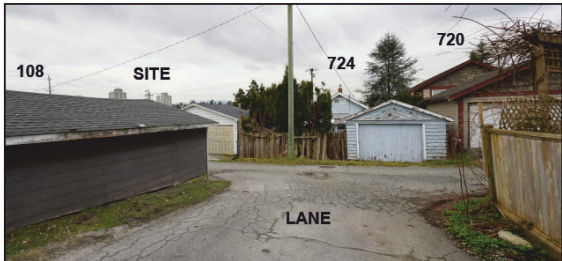
PHOTO 9: IN LANE LOOKING NORTH-EAST
