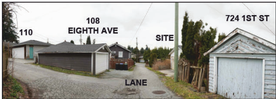
PHOTO 10: IN LANE LOOKING NORTH-WEST
