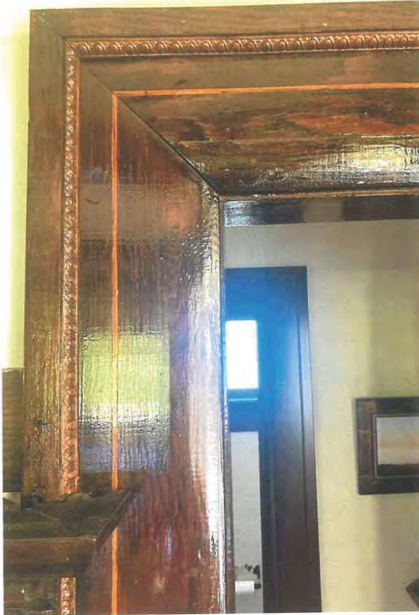
Main Floor Principal Rooms: Maple Inlaid Baseboard and Door and Window Trim Main Floor
