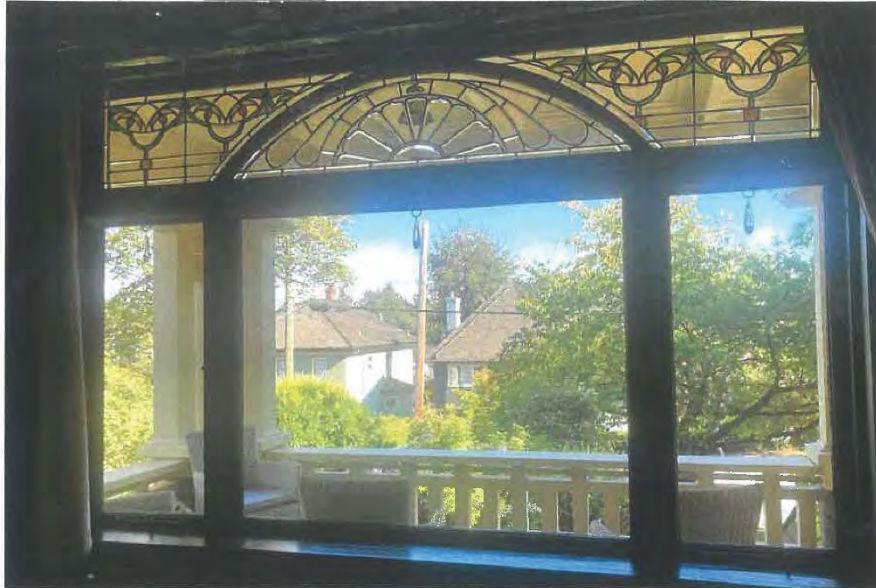
Living Room: Front/South Leaded Stained Glass Stationary Transom Window
