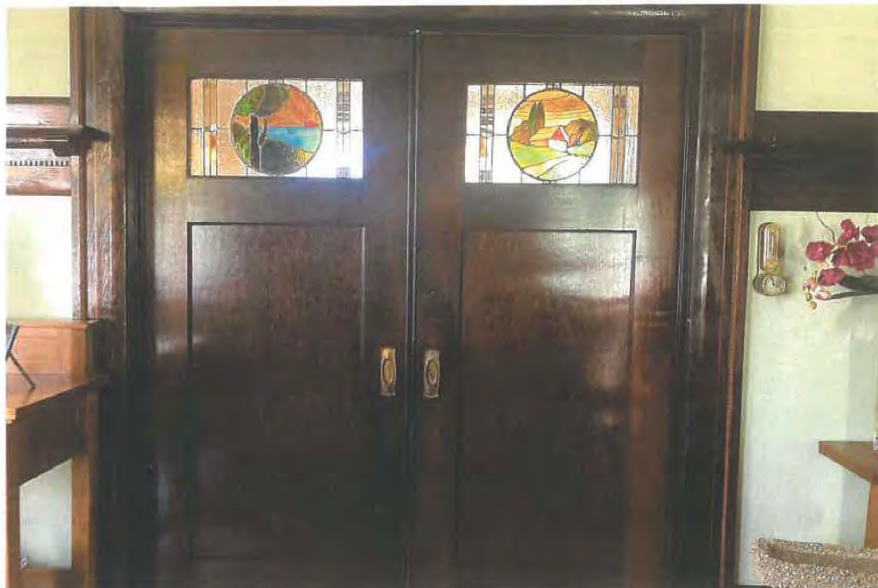
Pocket Doors: Inset Leaded Stained Glass Picture Panel between Dining Room and Living Room
