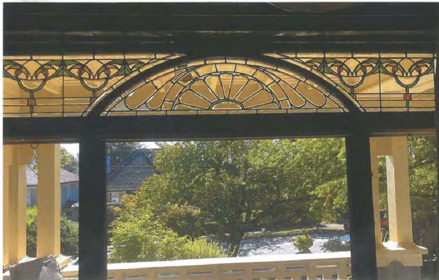
Living Room: Front/South Leaded Stained Glass Stationary Transom Window:
