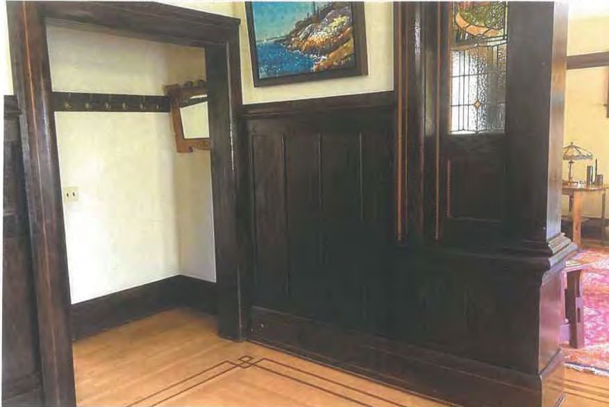
Main Floor Principal Rooms: Maple Inlaid Baseboard and Door and Window Trim Main Floor
