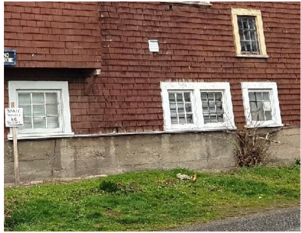
Above: interior (left) and exterior (right) photographs of the board-formed concrete foundation.
