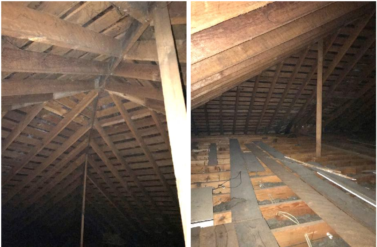
Above: photographs of the attic space showing the well constructed, dry roof structure and second floor ceiling beams.
