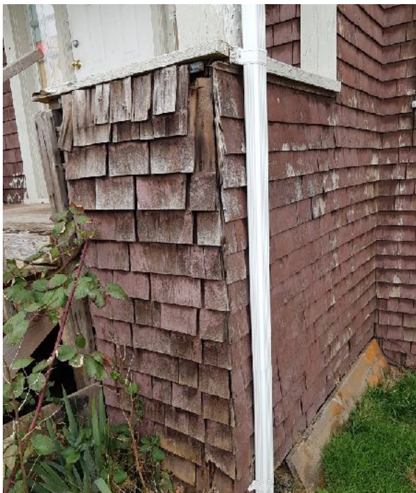
Above: front porch shingles (left) in the worst condition and north elevation (right) shingles in good condition.
