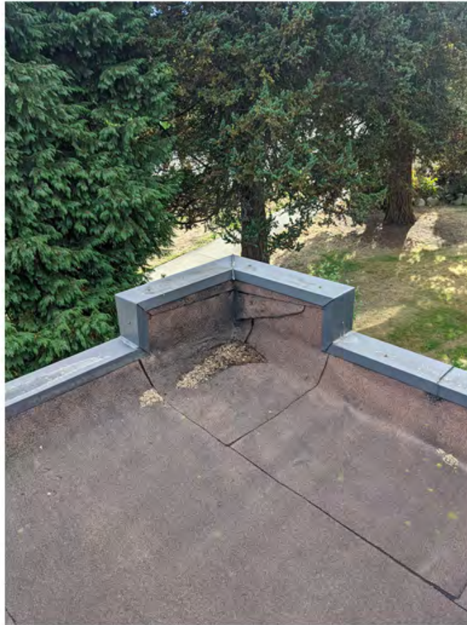
rolled asphalt seams degraded.jpg
