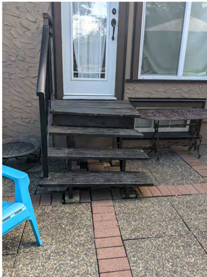
unit 351 - settlement in north entryway stairway.jpg
