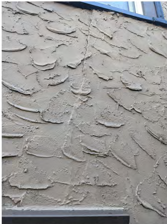
recently opened crack in stucco on east wall above crawl space access door.jpg
