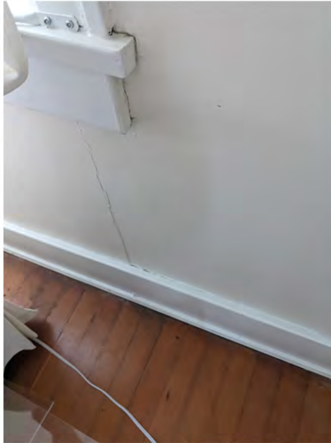
unit 351 - evidence of foundation settlement on south wall below window on main level.jpg
