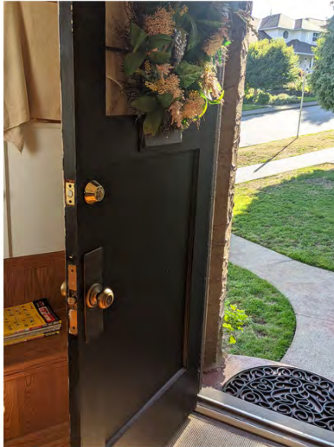
unit 349 - south doorway needs to be replaced due to settlement and faulty hardware.jpg
