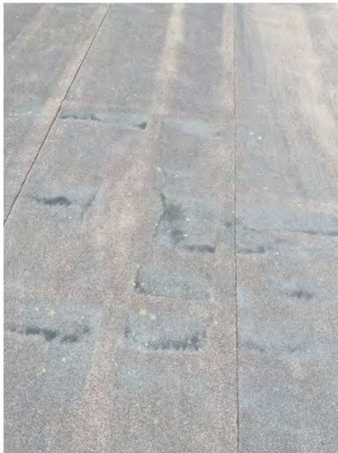
roof surface with degraded granular material.jpg
