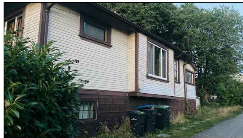
EXISTING HOUSE AT SIDE LANE
