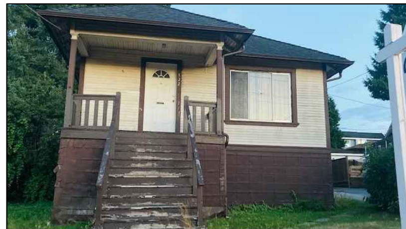
EXISTING HOUSE AT FRONT STREET
