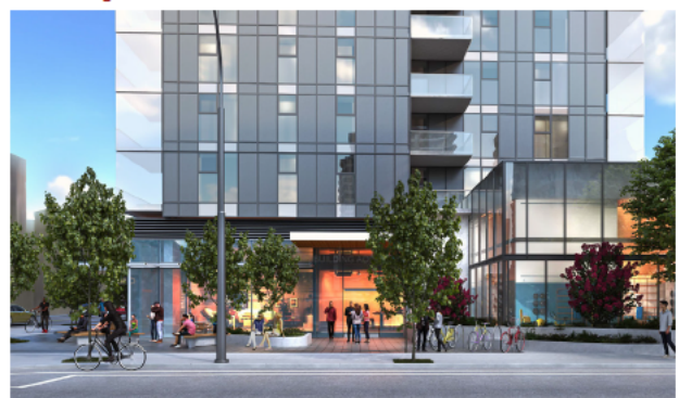
Entrance along Seventh Avenue
