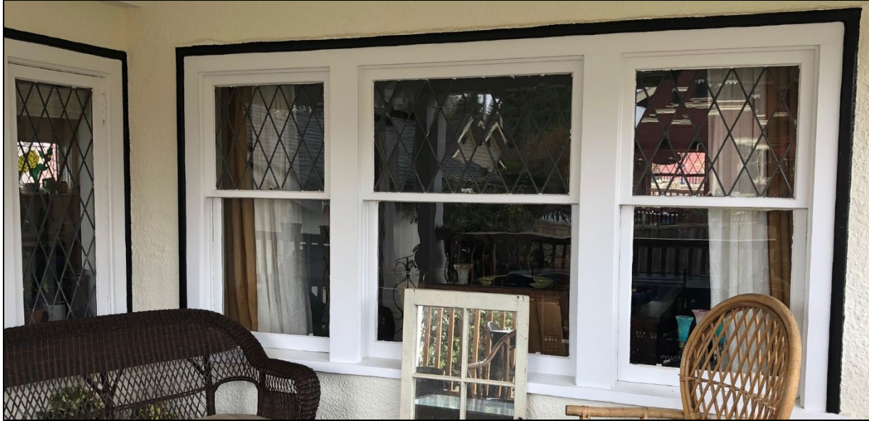
Fig. 22: The back deck of Edgar House at 323 Regina Street, 2020, illustrating the good condition of its original windows, with diamond patterned panes. (Source: Holisko)
