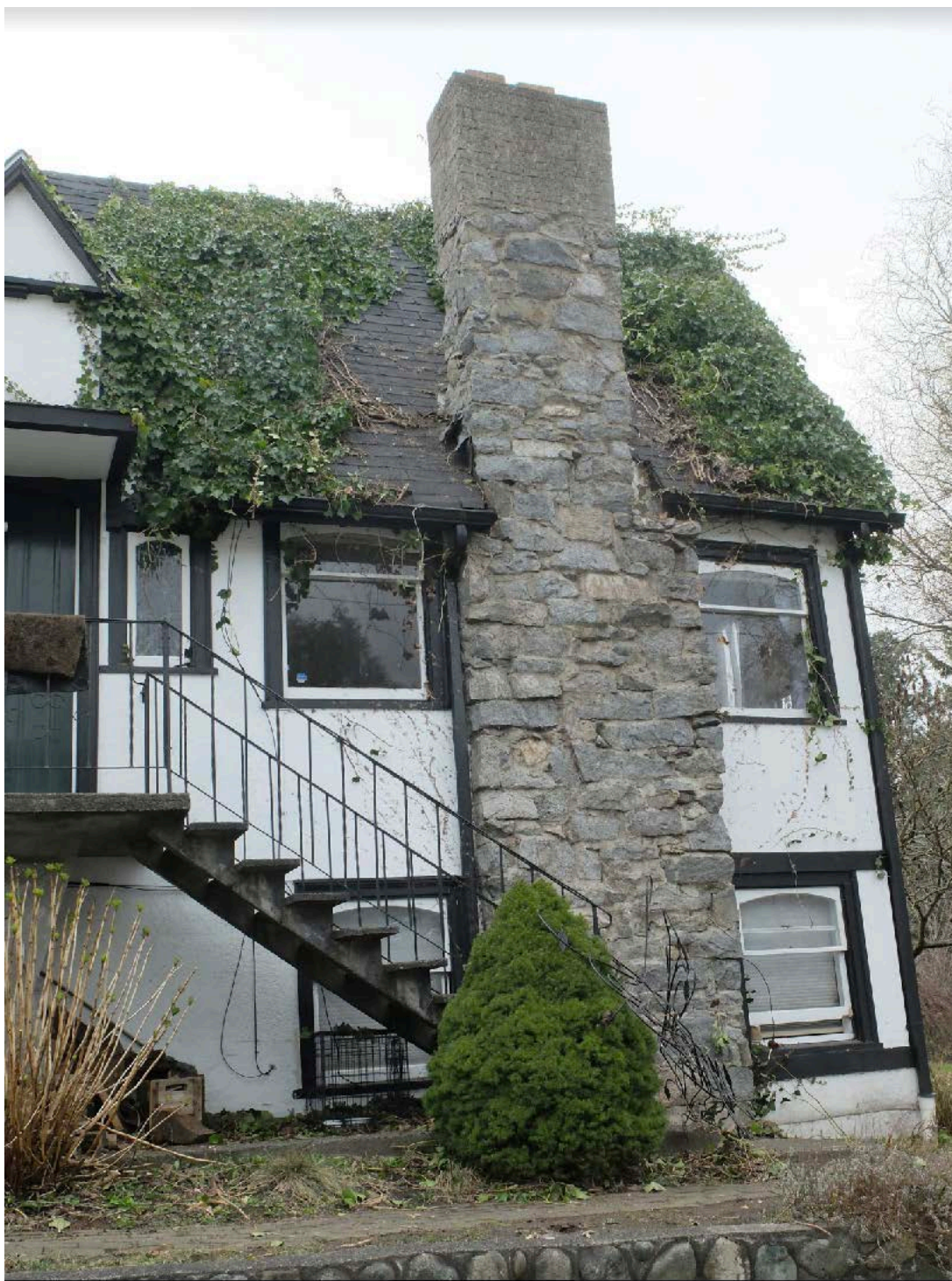
1st Street granite & concrete brick top chimney exposed after vine removal in early 2021.
