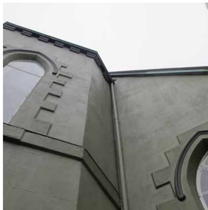
Exterior cement parging.
