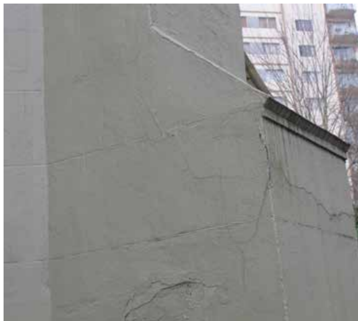
Cracking cement parging on buttress.
