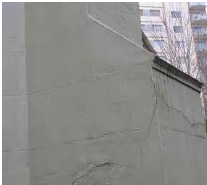
Cracking cement parging on buttress.
