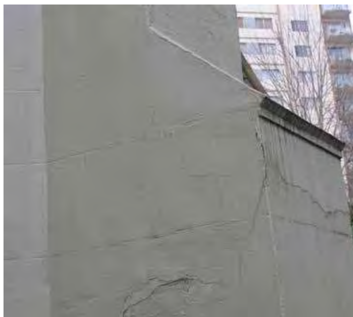
Cracking cement parging on buttress.
