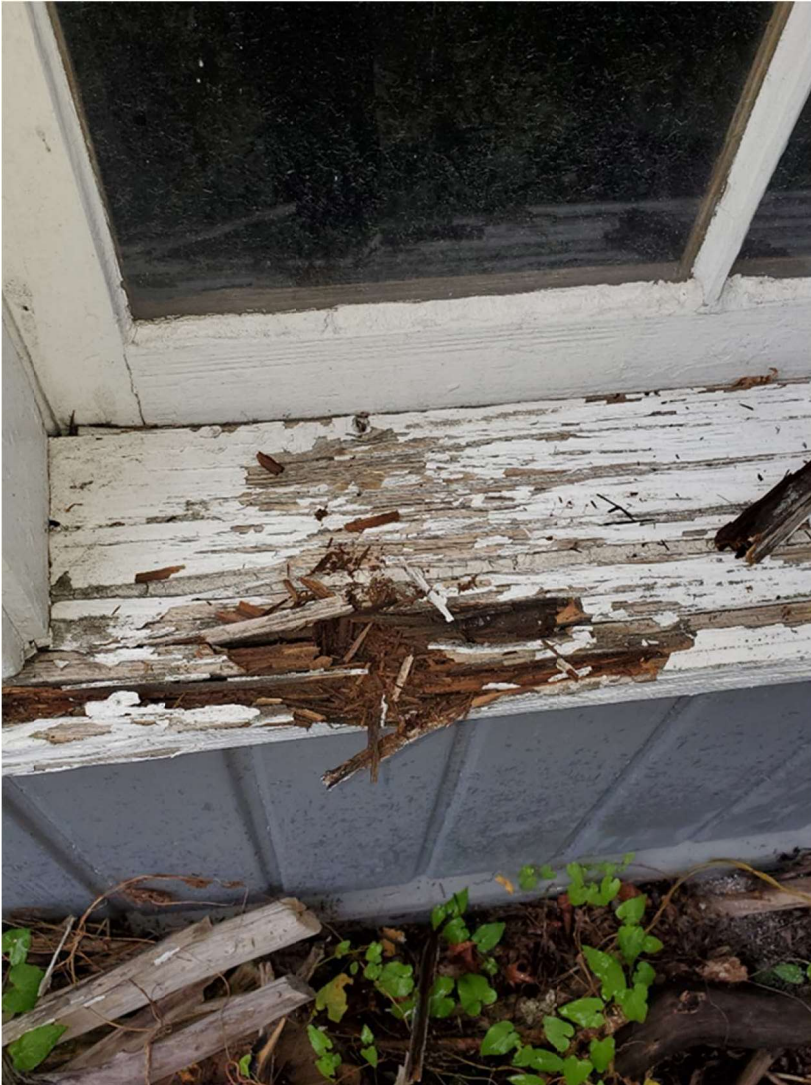
416 most wood windows beyond repair, fully decayed
