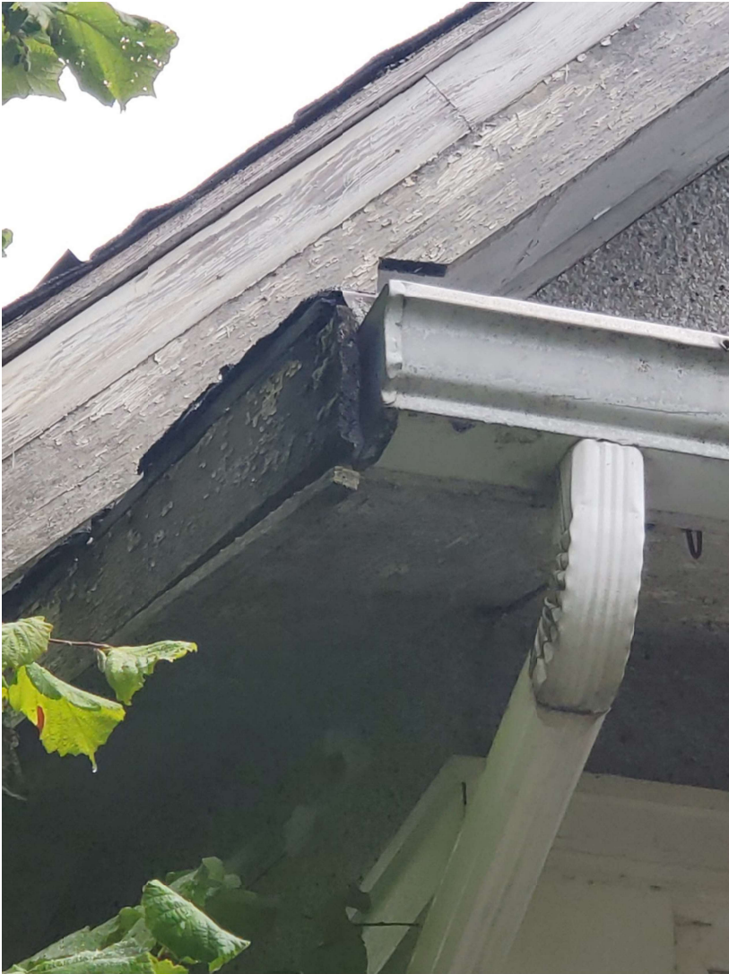
849 Roof eaves rotten and high potential of mold and structural damage
