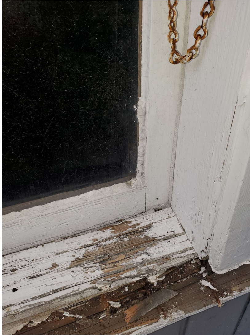
439 most wood windows beyond repair, fully decayed
