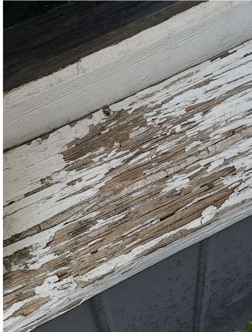
503 most wood windows beyond repair, fully decayed
