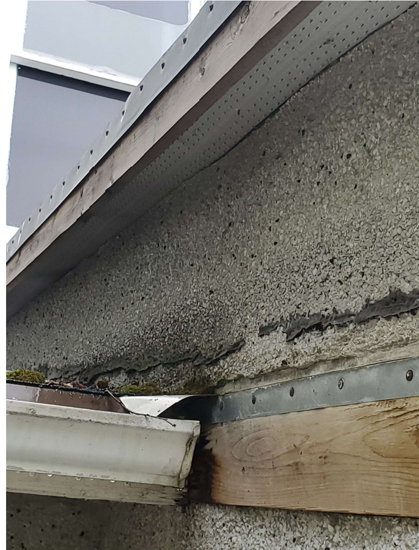
926 poorly maintained roof edges, high chance of internal water damage
