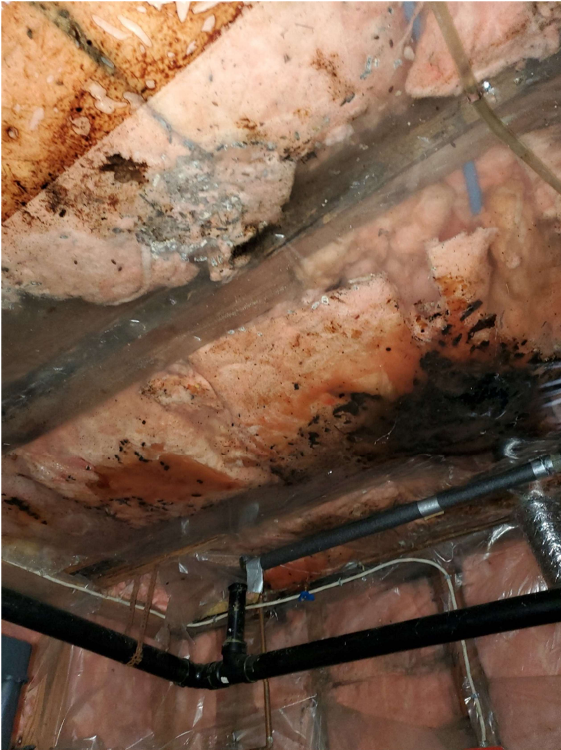
037 active water damage evident in basement along with mold
