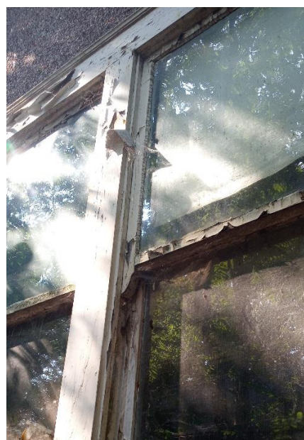
Figure 37: Double-hung window with sash horn
