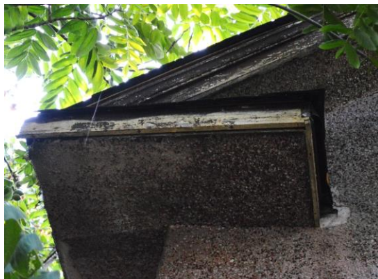
Figure 12: Gable end's return with stucco finish
