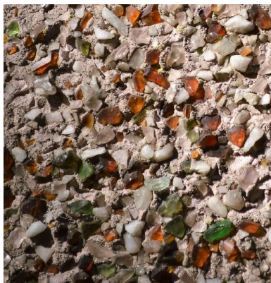
Figure 11: Bottle Dash Stucco detail
