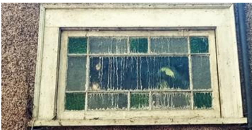
Figure 38: East side multipaned piano window with colour glass
