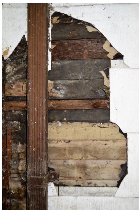
Figure 29: Cove lap siding below board underlay; the original siding is missing; the lower left are traces of cedar shingles
