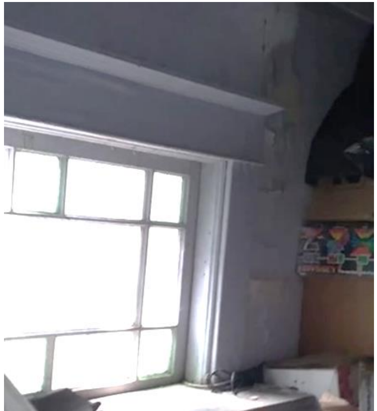
Figure 8: Interior multi-pane window and casing (Owner's photo)
