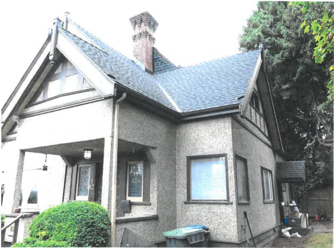
northeast corner view
