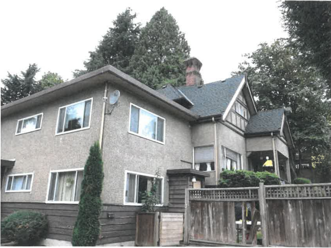
southeast corner view
