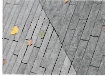
Ground floor materials / pavers
