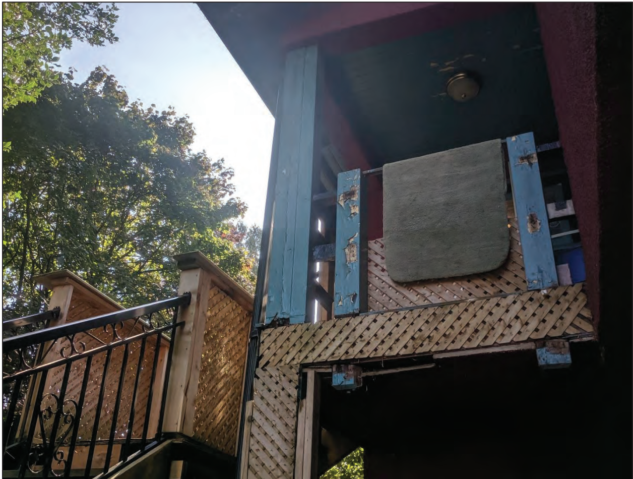
Fig. 15: Southeastern view of the back of Henderson House at 112 Royal Avenue, 2019, illustrating some of the deterioration of the house's back porch. (Source: Cummer)
