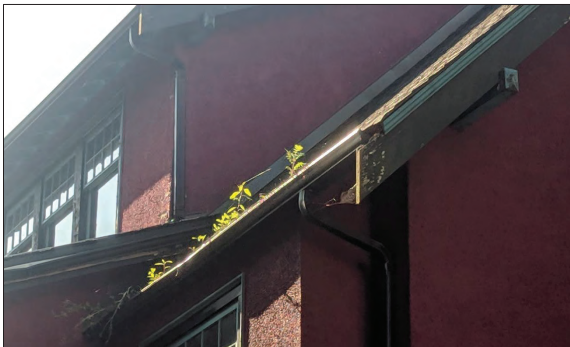
Fig. 17: Southeastern view of Henderson House at 112 Royal Avenue, 2019, illustrating another fascia board deterioration as well as additional plant growth in the house's gutters. (Source: Cummer)
