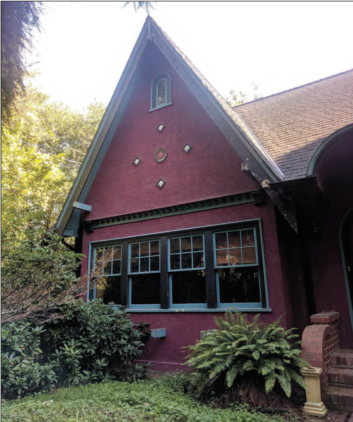
Fig. 9: Partial front view of Henderson House at 112 Royal Avenue, 2019, illustrating the steeply pitched offset front gable with ornamental diamond detailing, floral roundel and small arched window at the top as well as the dentil moulding, with a partial view of the arched roofline over the front door and the arched brick front stairs. Note the surviving window box supports, although the window boxes themselves are missing. (Source: Cummer)
