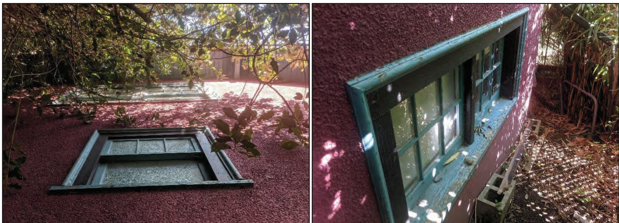
Figs. 22 and 23: Left (Fig. 22) shows a frosted double-hung, divided-light wood window along the western side of the building. Right (Fig. 23) shows a lower window along the same side with visible paint peeling. (Sources: Cummer)
