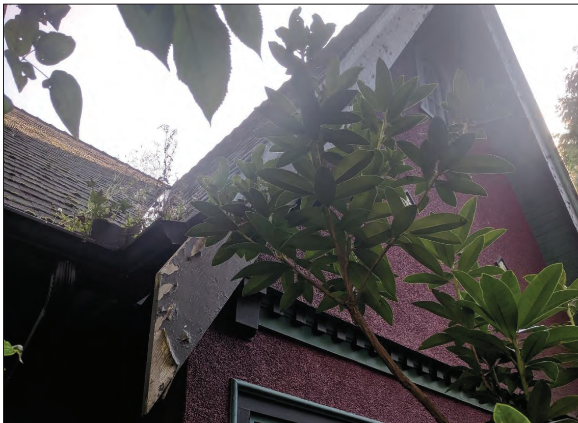
Fig. 16: Northeastern view of Henderson House at 112 Royal Avenue, 2019, illustrating the roof fascia deterioration in the front offset gable, as well as some plant growth in the house's gutters. (Source: Cummer)
