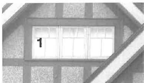
1 gable triple-assembly window
