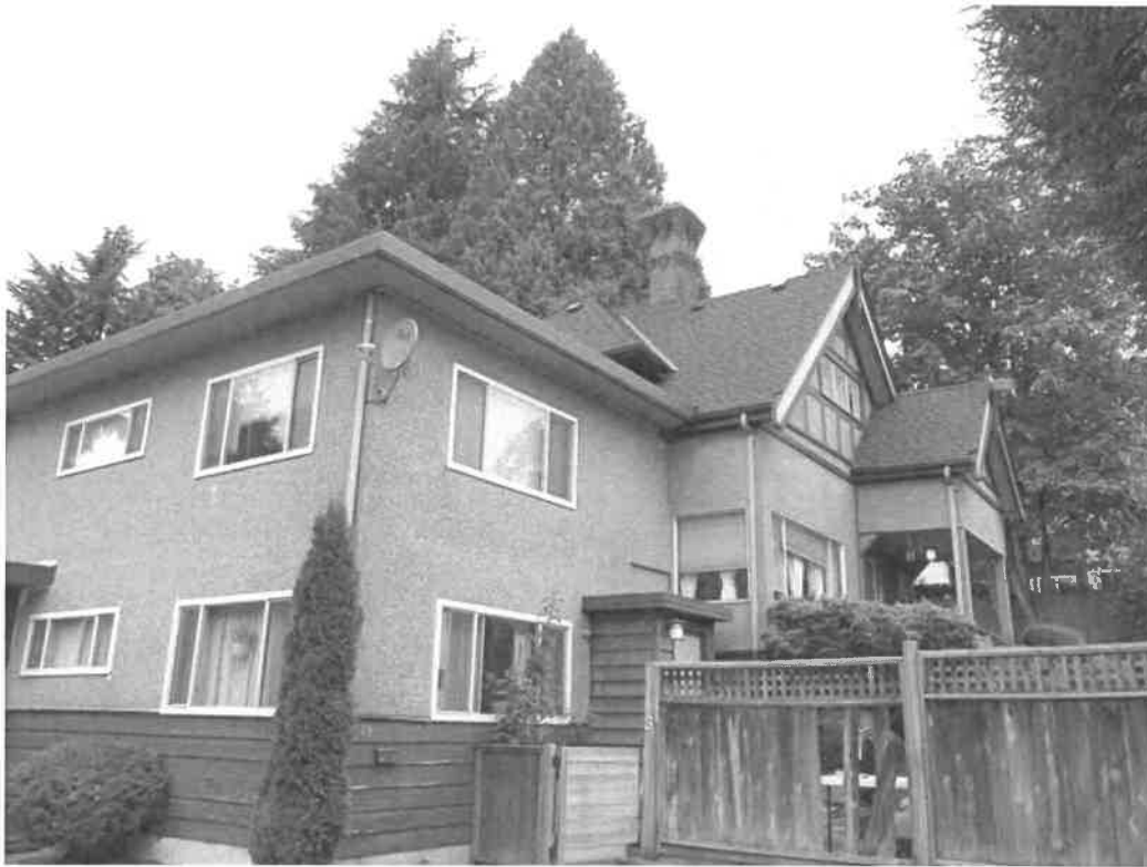
southeast corner view
