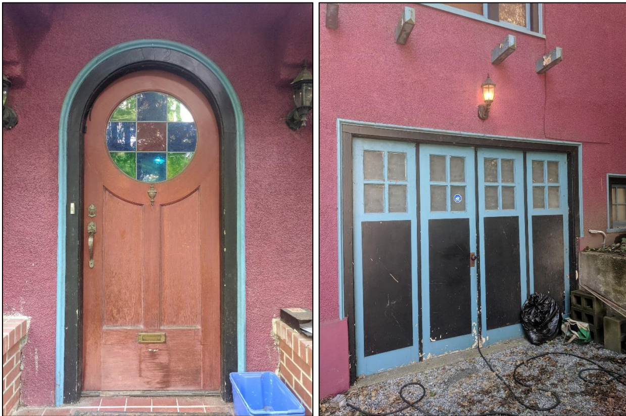
Figs. 27 and 28: Left (Fig. 27) shows the front door of Henderson House at 112 Royal Avenue, 2019, illustrating its largely good condition, minus some weathering at the bottom of the door, along with its intact, multi-coloured stained-glass window. Right (Fig. 28) shows the four-panel set of doors along the eastern façade of the house. It is also in good condition, minus some paint peeling near the bottom of some of the panels. (Sources: Cummer)
