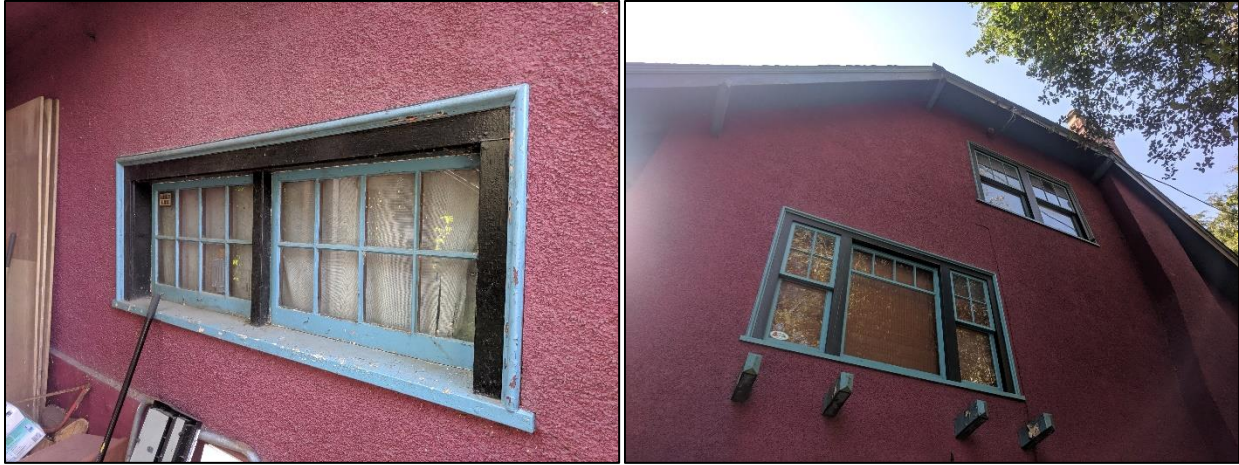
Figs. 25 and 26: Left (Fig. 25) shows a divided-light wood window at the back of Henderson House at 112 Royal Avenue, 2019, illustrating some deterioration. Right (Fig. 26) shows the eastern side of the property and its double-hung, divided-light wood windows. Again, note the supports for the missing window boxes. (Sources: Cummer)
