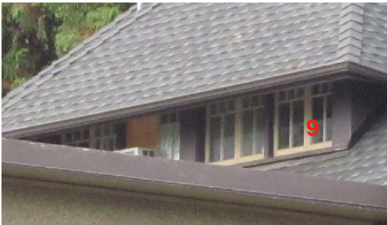
9 dormer double assembly windows. One sash is missing where an air conditioning unit was installed.
