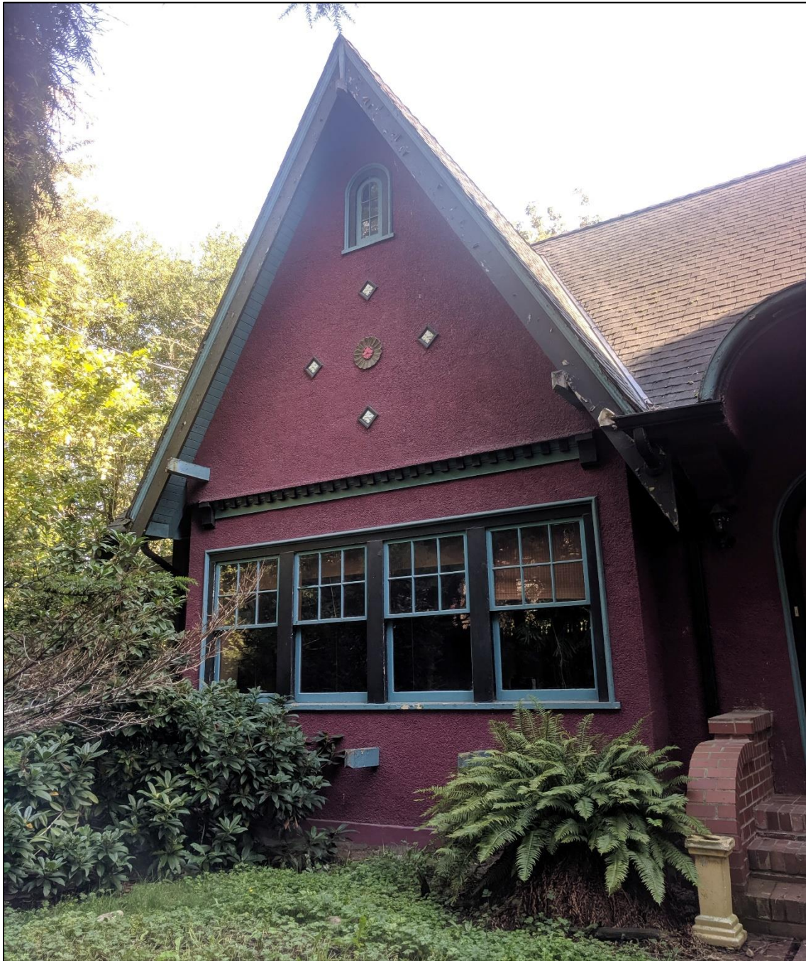
Fig. 9: Partial front view of Henderson House at 112 Royal Avenue, 2019, illustrating the steeply pitched offset front gable with ornamental diamond detailing, floral roundel and small arched window at the top as well as the dentil moulding, with a partial view of the arched roofline over the front door and the arched brick front stairs. Note the surviving window box supports, although the window boxes themselves are missing. (Source: Cummer)
