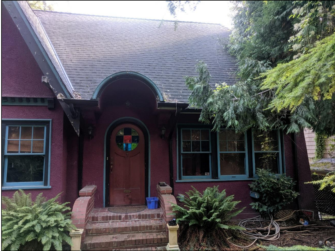
Fig. 10: Partial front view of Henderson House at 112 Royal Avenue, 2019, highlighting the arched roofline over the arched front door with multi coloured stained glass window and the arched brick front stairs, as well as some of the double-hung divided-light wood windows. (Source: Cummer)
