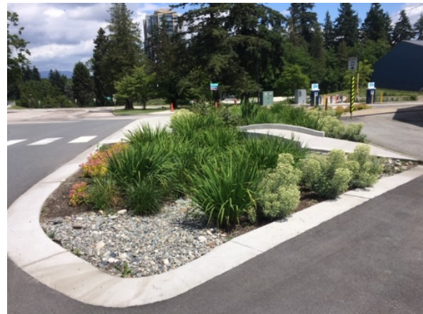
Photo 41 A rain garden installed at Queens Park
