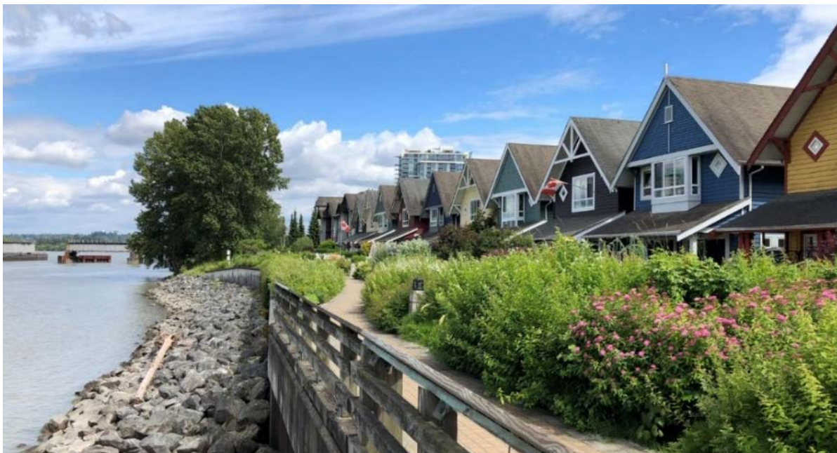
Photo 3 Recent Fraser River foreshore development in Queensborough (DHC)
