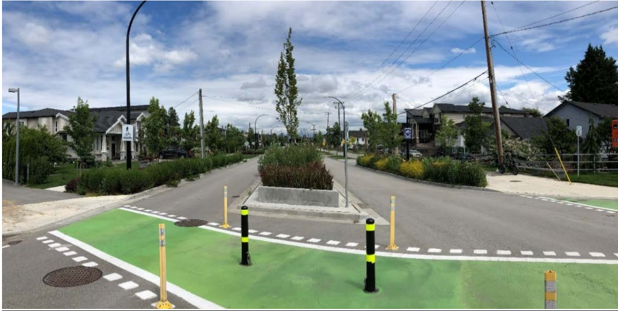
Photo 29 Centre median and boulevard plantings recently installed at Ewen Ave and Boundary road in Queensborough
