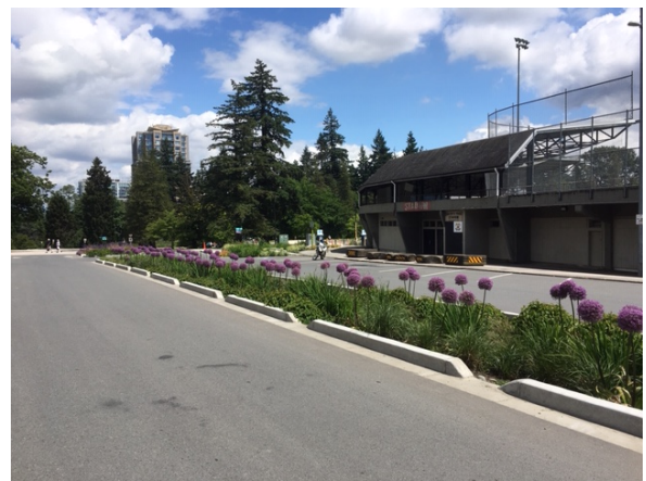
Photo 43 A rain garden installed in a new parking lot in Queens park.
