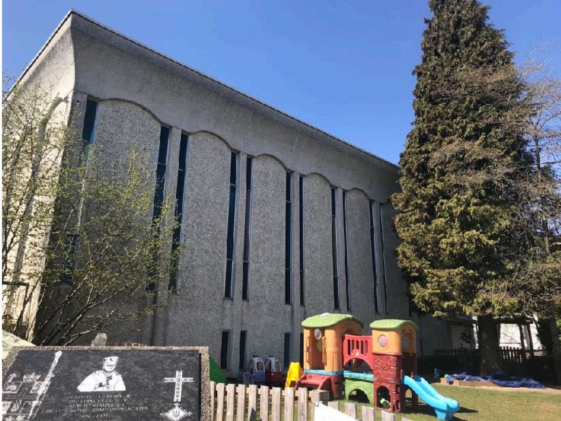
Side view (facing 5th Street)
