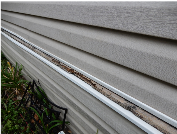
Exposed deteriorating trim board.
