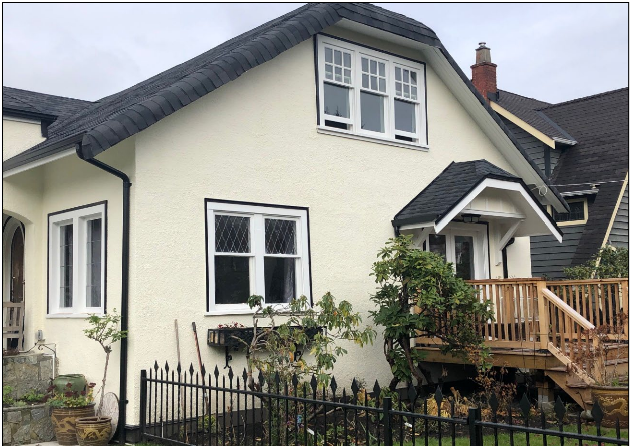
Fig. 14: Eastern corner view of Edgar House at 323 Regina Street, 2020. (Source: Holisko)
