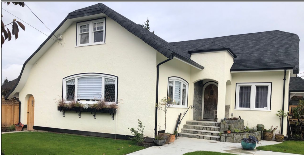
Figs. 17a and 17b: Comparative views of Edgar House at 323 Regina Street, 2019 (top) and 2020 (bottom), illustrating the various work done on site, listed in full on the following page. (Sources: Vallee (top) and Holisko)
