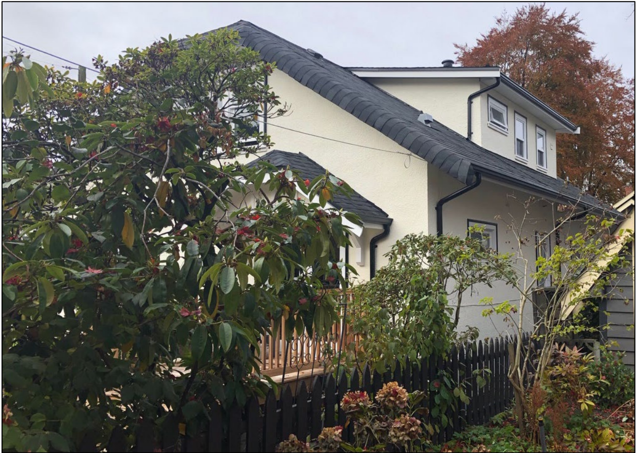
Fig. 15: Northeastern side of Edgar House at 323 Regina Street, BC, 2020. (Source: Holisko)
