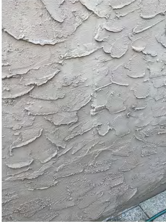
crack in stucco on east wall just north of lower level crawl space door.jpg
