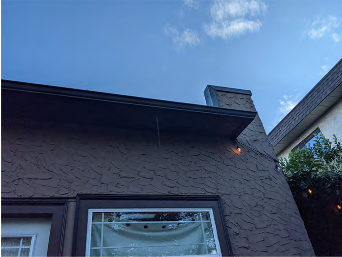
unit 351 - north wall upper level on west side.jpg
