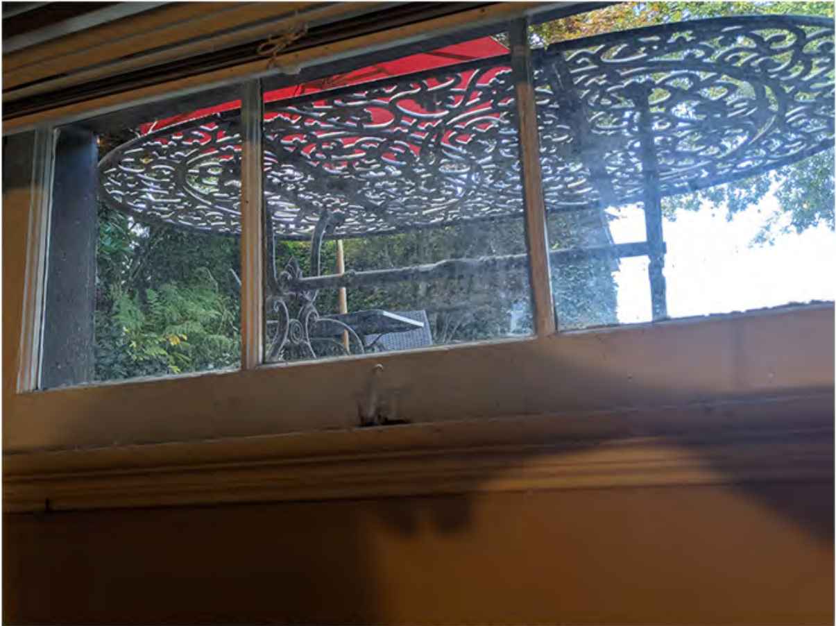
unit 351 - wood framed window in lower level.jpg
