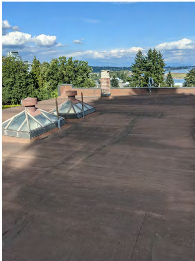
WC skylights for both units.jpg
