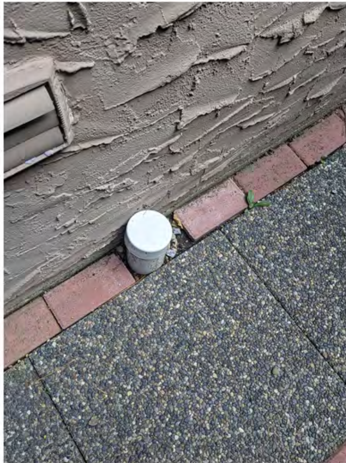
unit 351 - weeping tile clean-out on west outer wall.jpg
