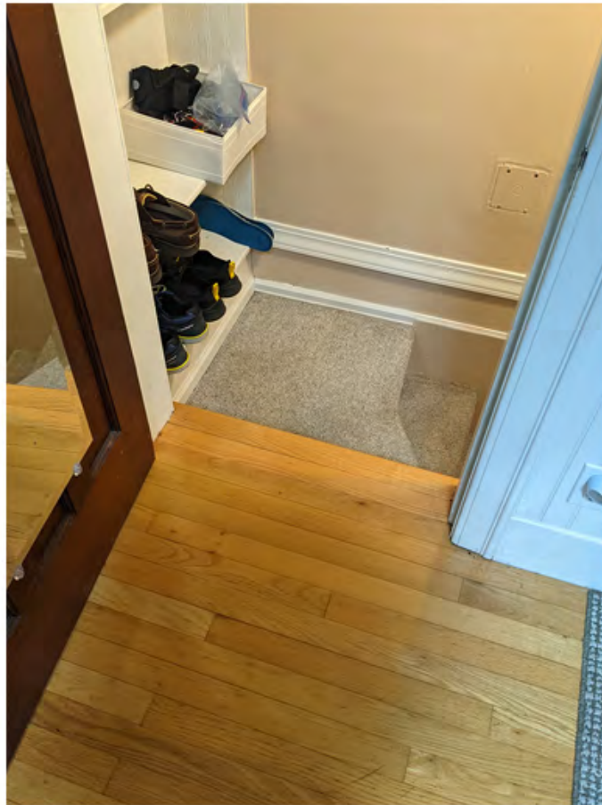
unit 351 - flooring in upper level and stairwell to lower level.jpg
