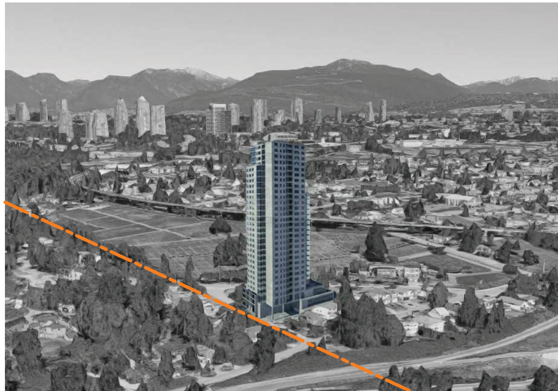
VIEW 2 - FROM SOUTH
