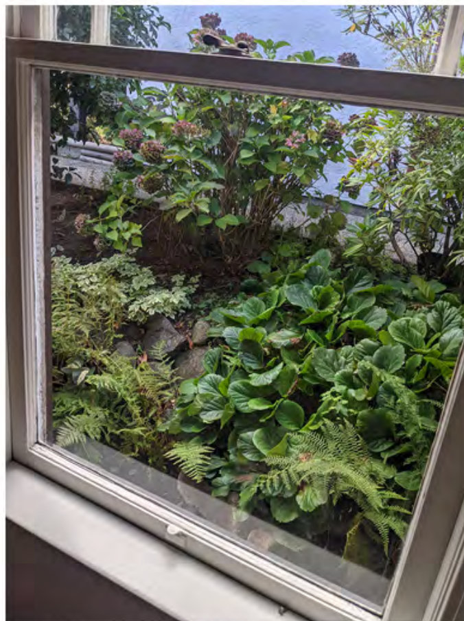
unit 351 - wood framed window in sitting area on west wall.jpg
