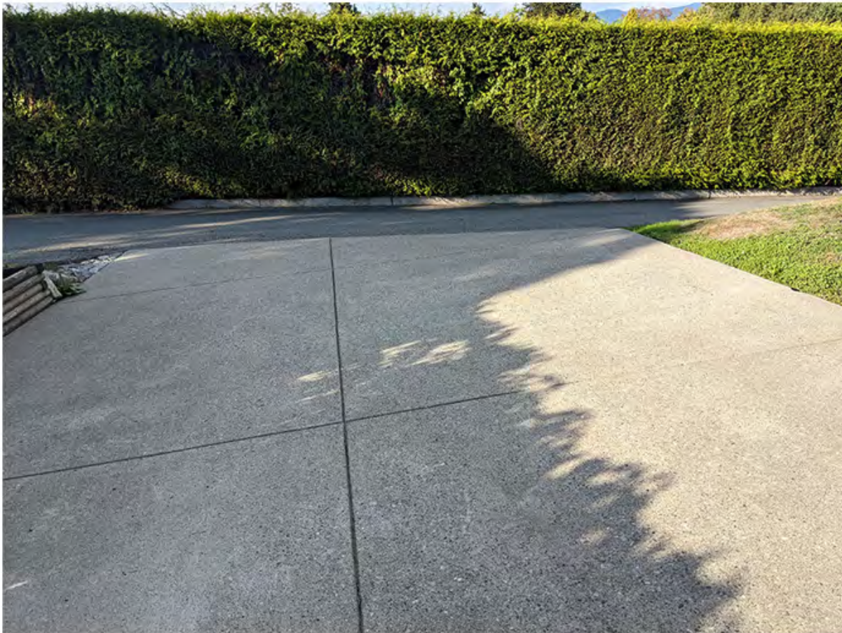
unit 351 - concrete parking pad on north side.jpg
