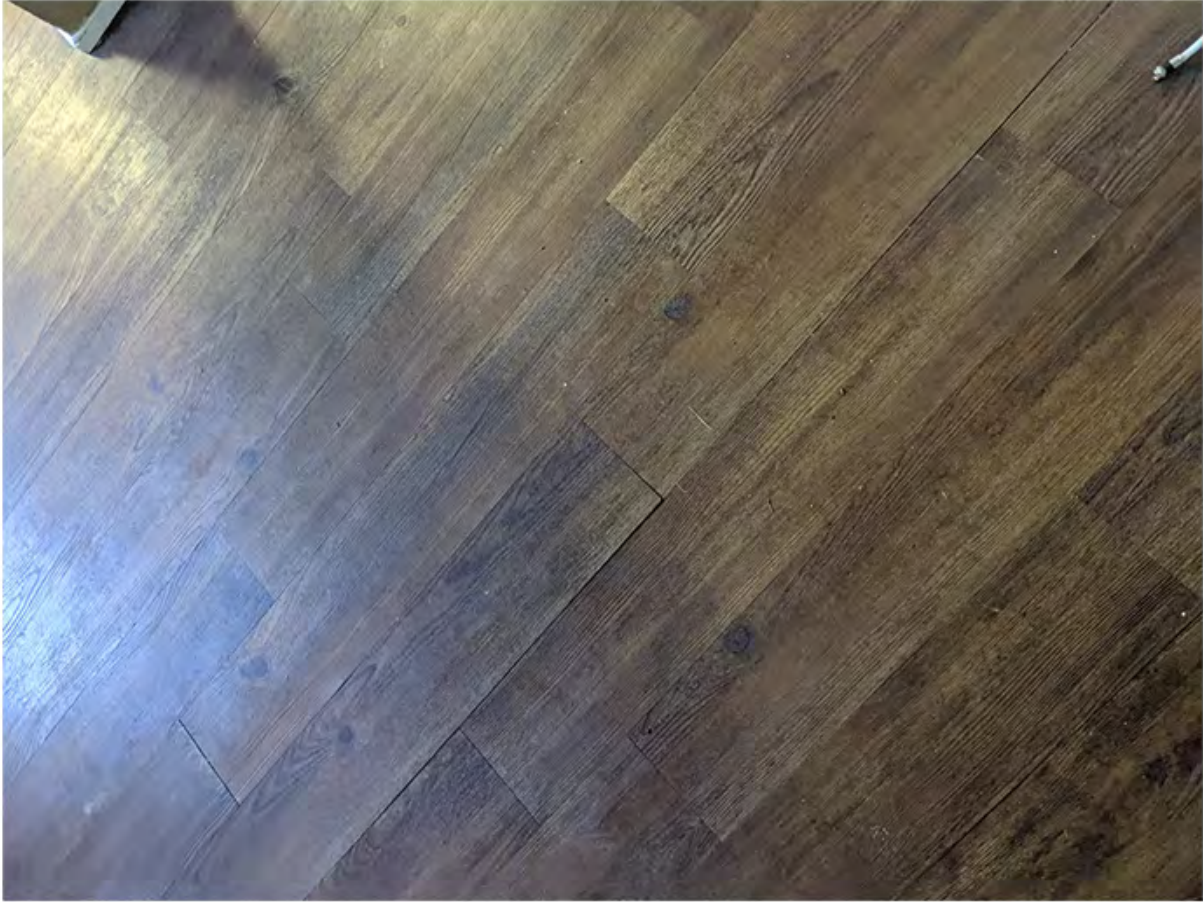
unit 349 - lower level flooring.jpg
