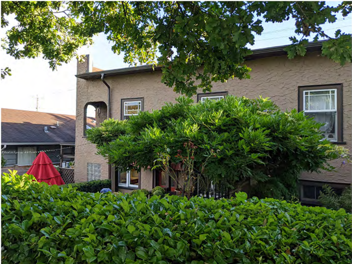
unit 349 - north wall.jpg
