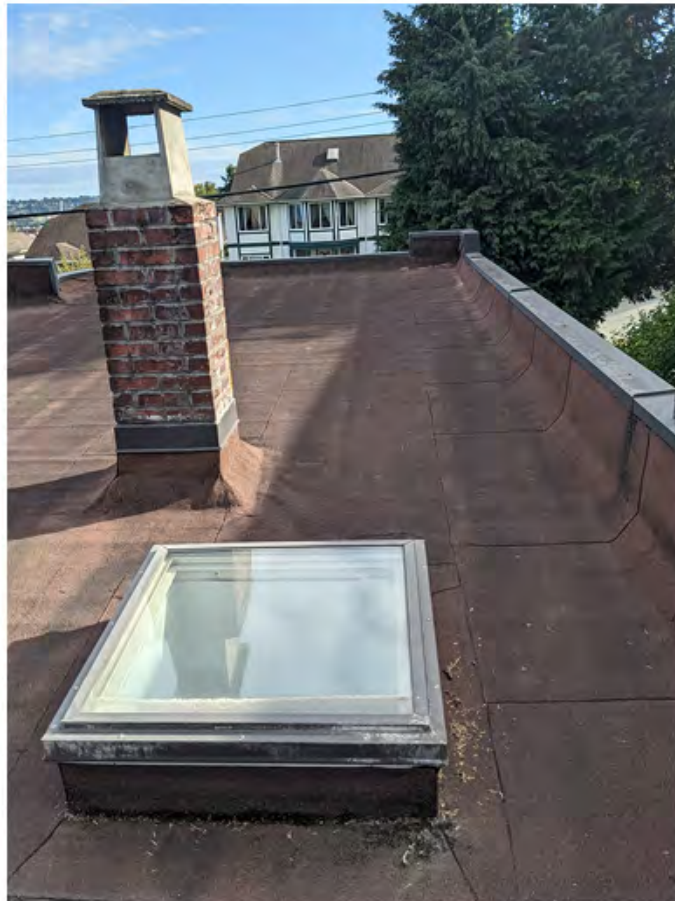
unit 351 kitchen skylight and chimney.jpg
