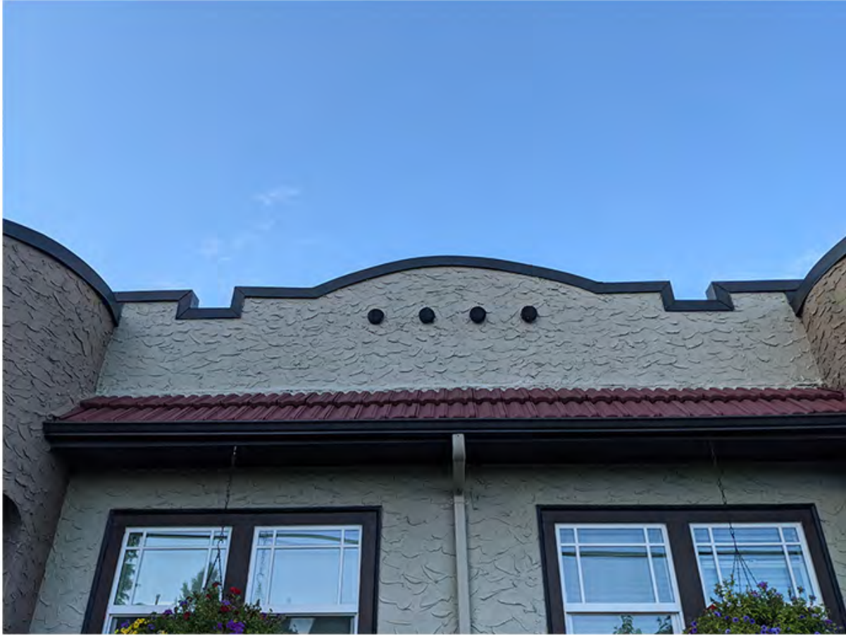
attic venting on south side.jpg
