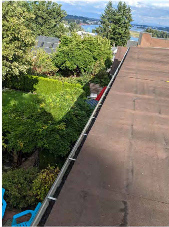
view looking east along north eavestrough.jpg
