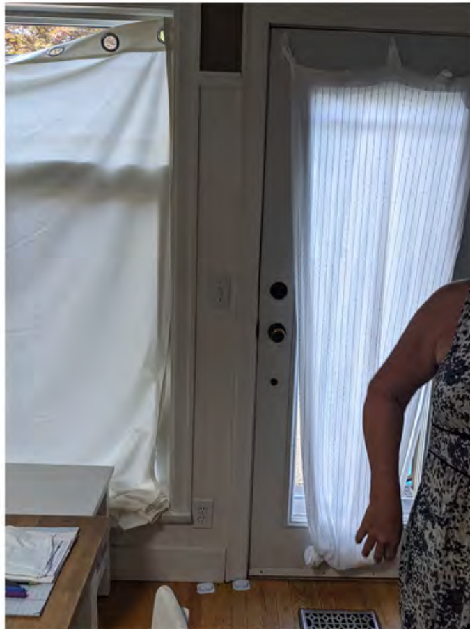
unit 351 - north entryway door.jpg
