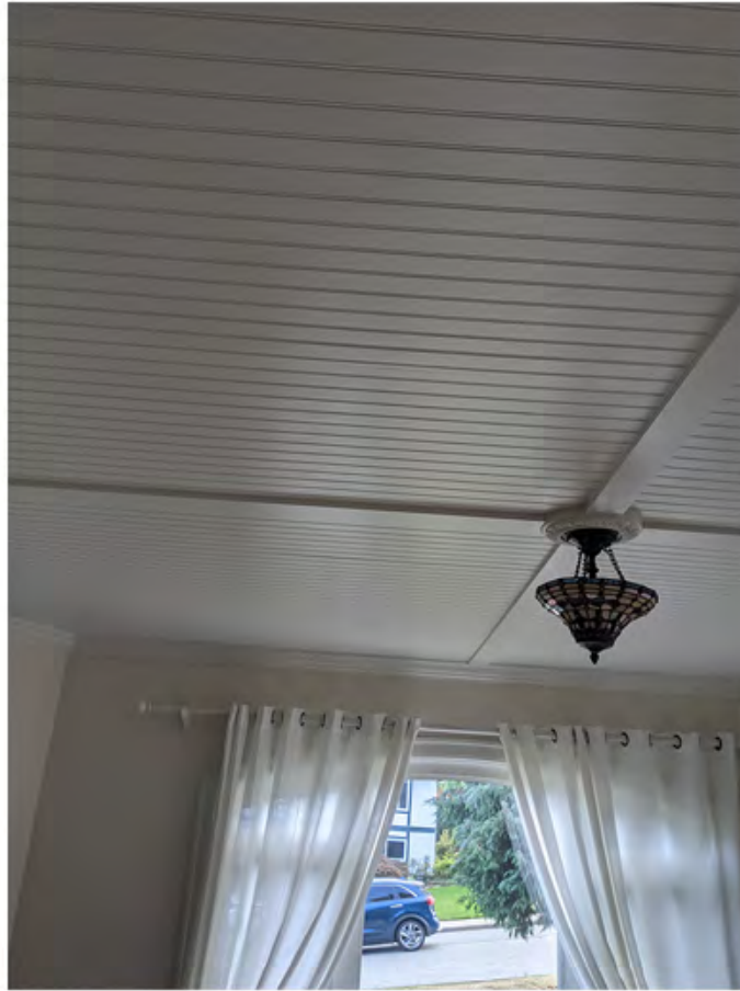
unit 351 - ceiling in sitting room.jpg
