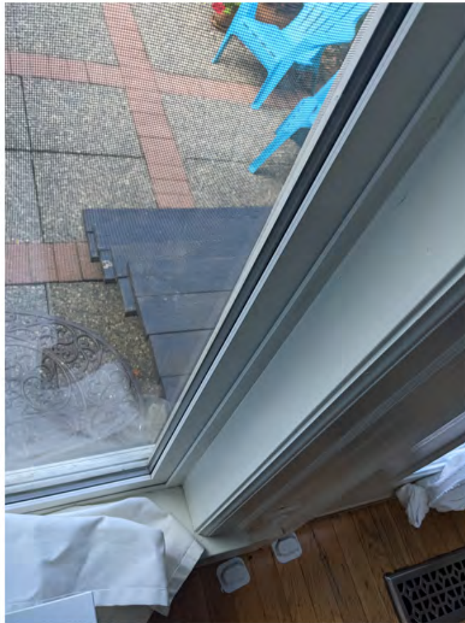
unit 351 - PVC framed window in kitchen on north wall.jpg
