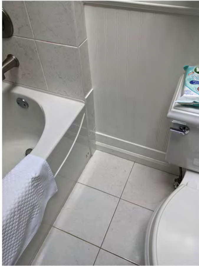
unit 351 - WC flooring wall and surround materials.jpg
