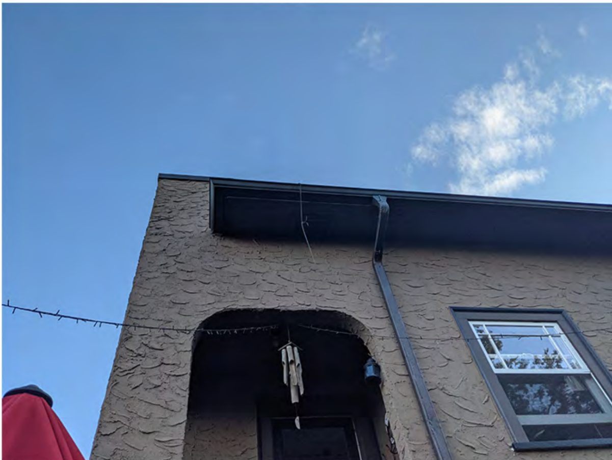
unit 349 - eavestrough downspout on north wall east side.jpg
