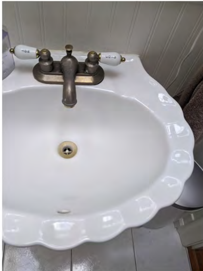
unit 351 - main level sink.jpg
