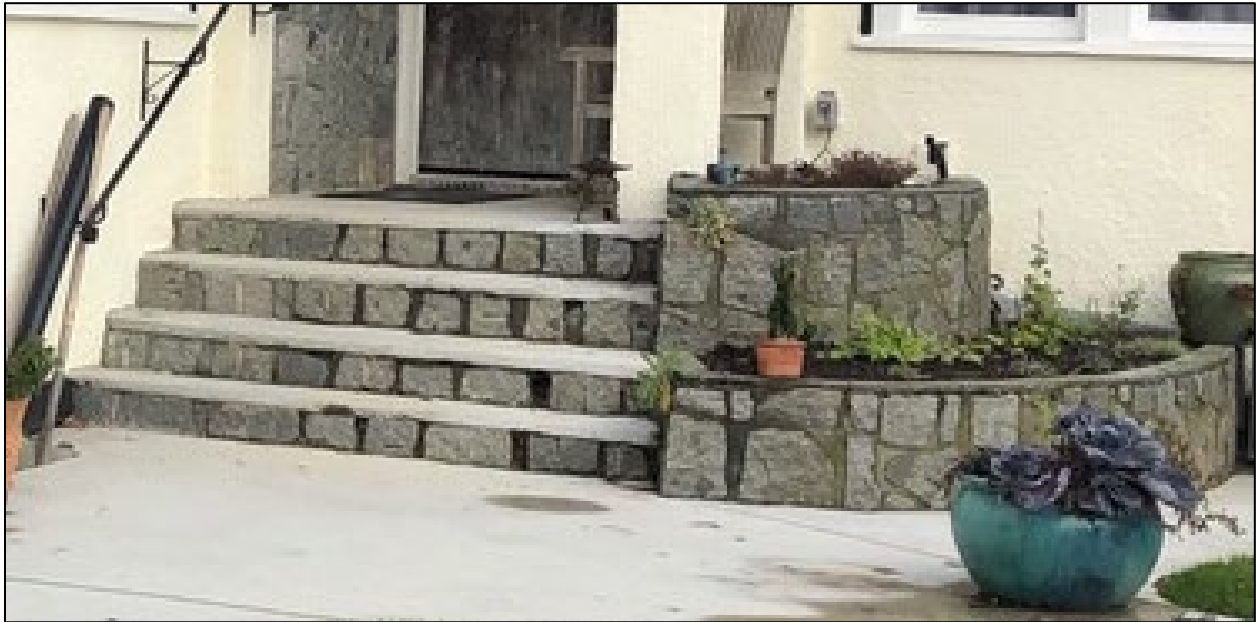
Fig. 18: Front stone steps and planter of Edgar House at 323 Regina Street, 2020, illustrating the minor maintenance concerns, such as moss growth and other plants growing between the stone slabs. (Source: Holisko)
