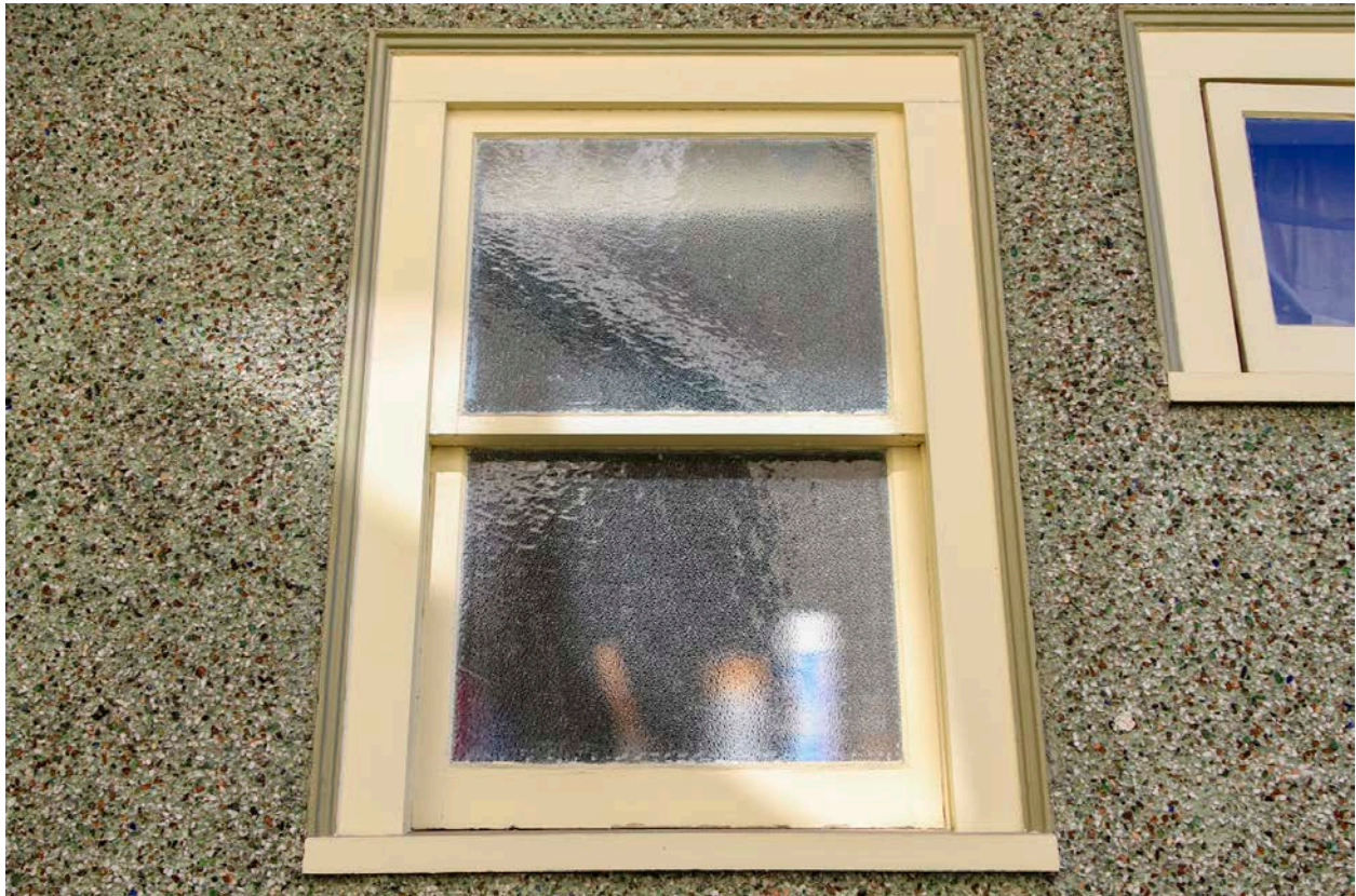
Detail of a 1-over-1 wood sash window on the northwest elevation of the Morrow Residence, Sept. 7, 2021.
