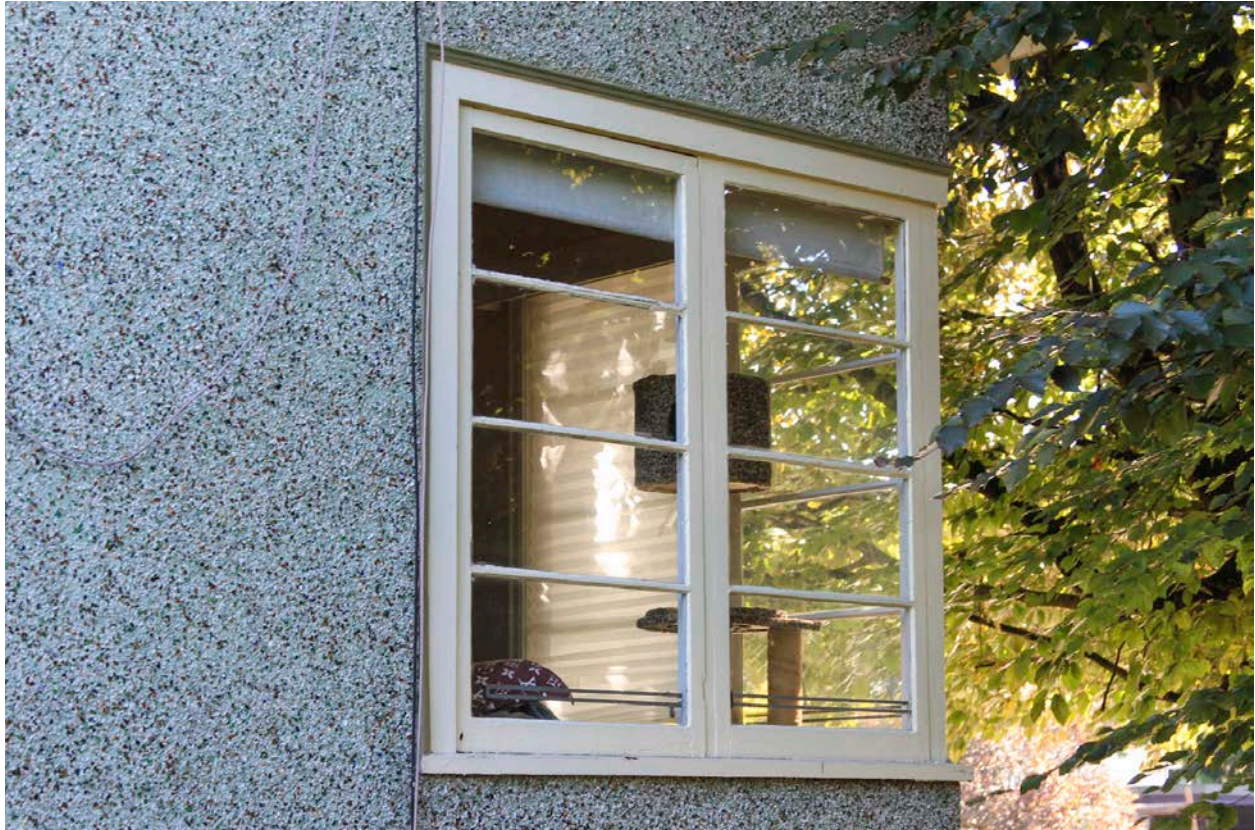
Detail of a multi-assembly corner wood sash window on the south corner of the Morrow Residence, Sept. 7, 2021.
