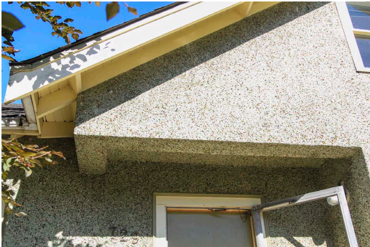
Detail of stuccoed soffit immediately above the recessed front entrance of the Morrow Residence, Sept. 7, 2021.
