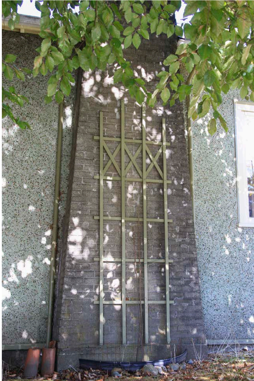
Detail of the base of the grey brick external tapered chimney on the front elevation of the Morrow Residence, Sept. 7, 2021.
