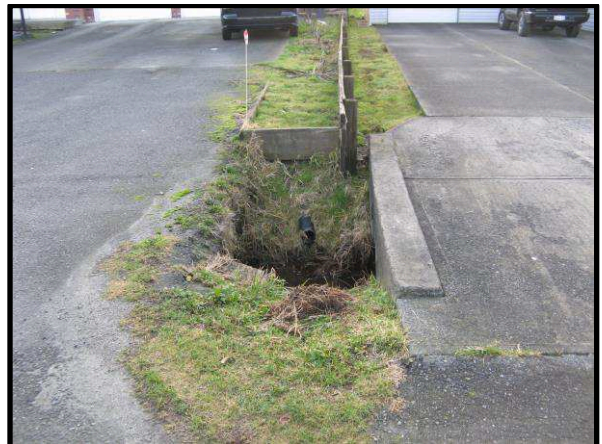
Unsafe gap b/n two immediate D/W crossings
