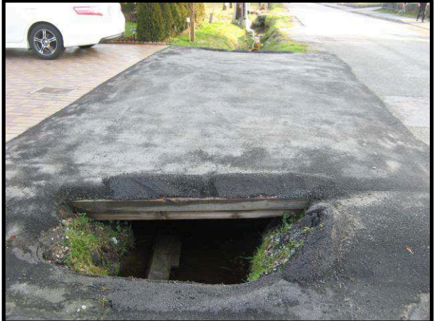
Existing unauthorized D/W culvert extensions
