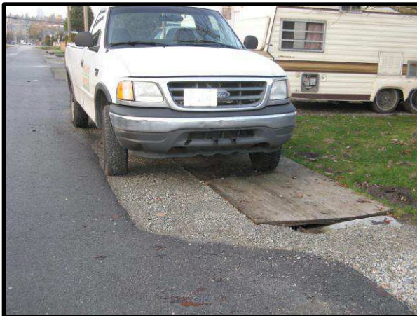
Existing unsafe plywood ditch cover
