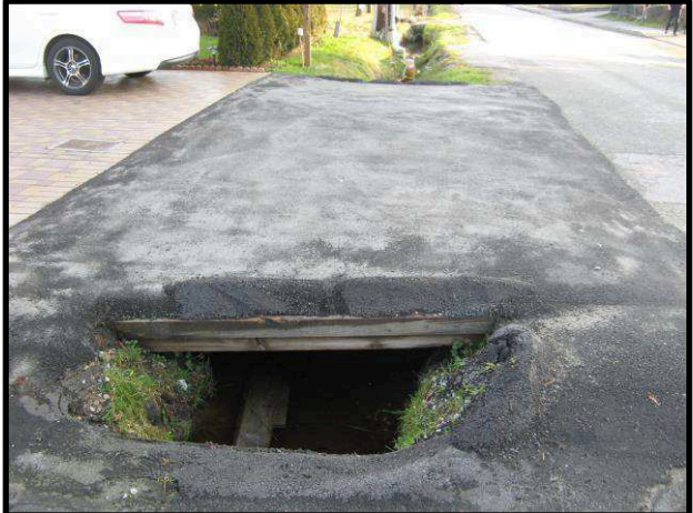
Existing unauthorized D/W culvert extensions
