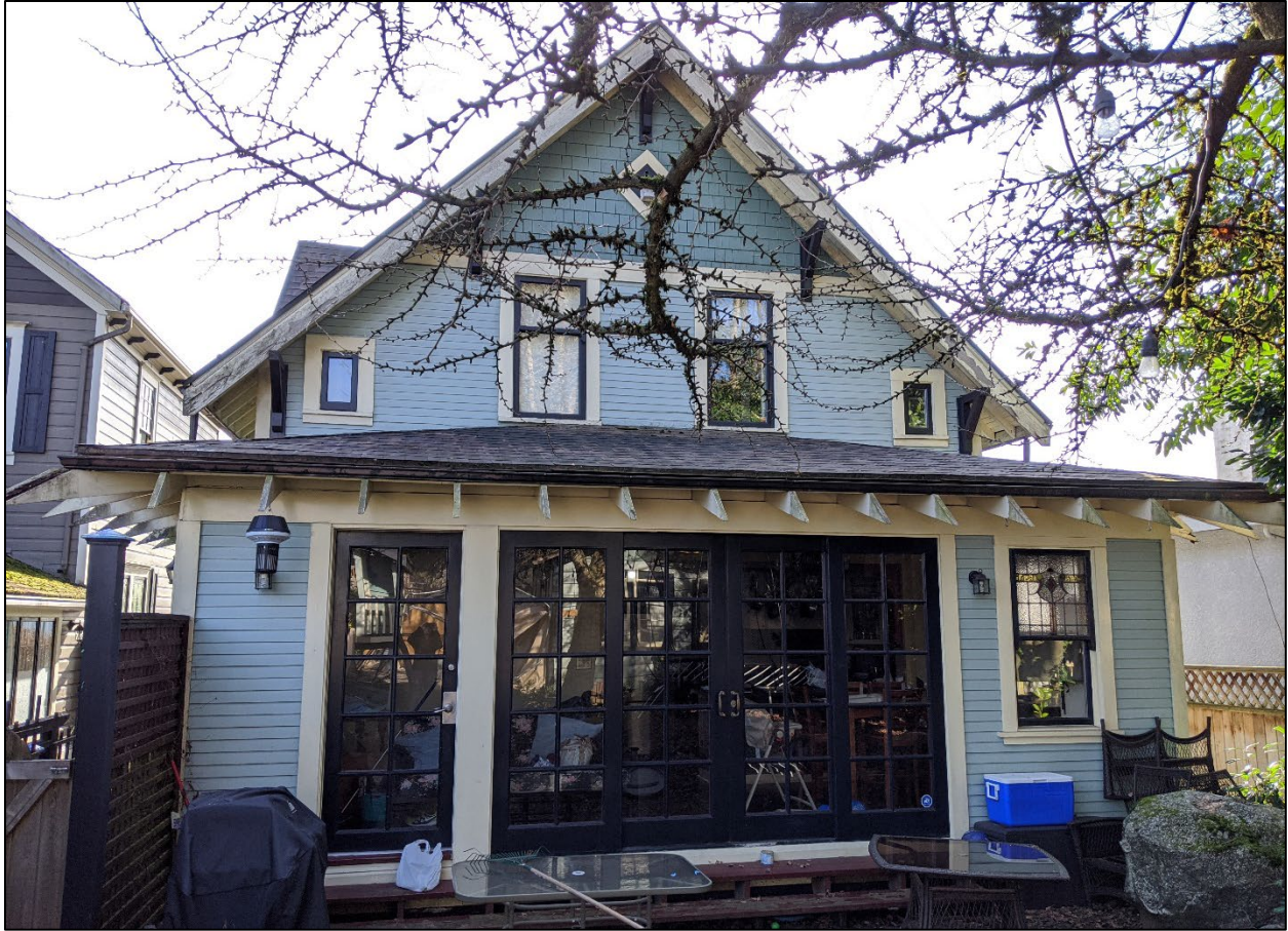
Fig. 8: Back view of Adams House at 515 St George Street. Note the brackets and range of windows, including a double hung horned stained-glass window on the right as well as two other double hung horned wood windows in the upper middle along with a diamond shaped window in the rear gable. (Source: Cumber)
