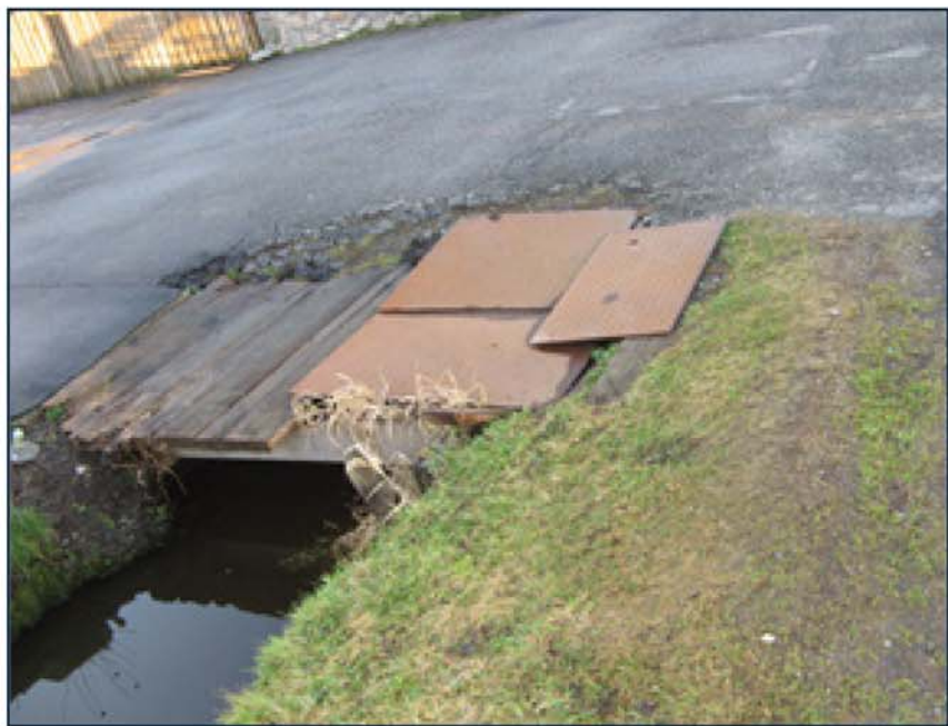
Existing non-standard rotten wood retaining wall.
