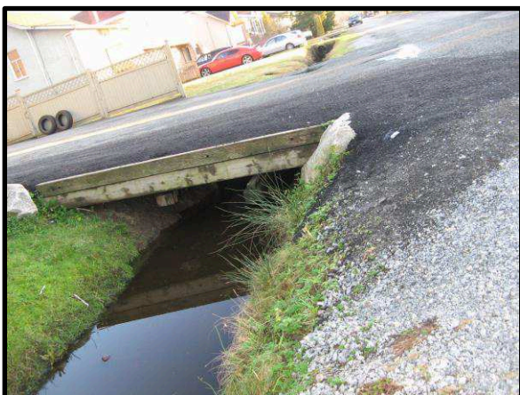
Existing unauthorized D/W crossing extension
