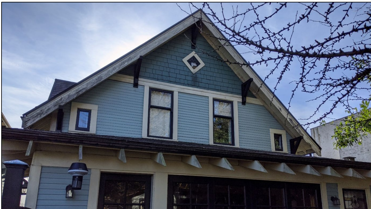
Fig. 11: Back gable of Adams House at 515 St George Street, showing the dirty rafter tails and soffits as well as the peeling fascia boards, in need of repainting. (Source: Cummer)
