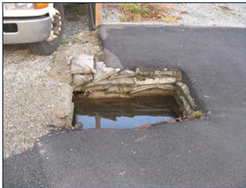
Existing hazardous gap between two driveway culverts.
