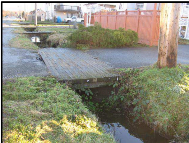
Existing non-standard wood cribbing
