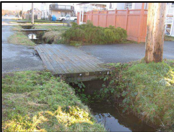
Existing non-standard wood cribbing
