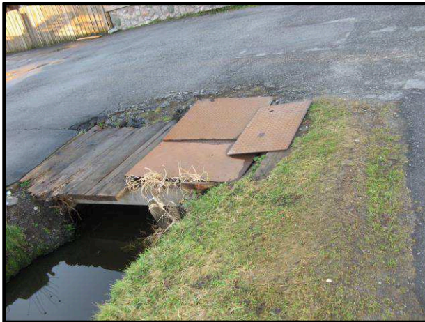
Existing unsafe pedestrian crossing ditch cover
