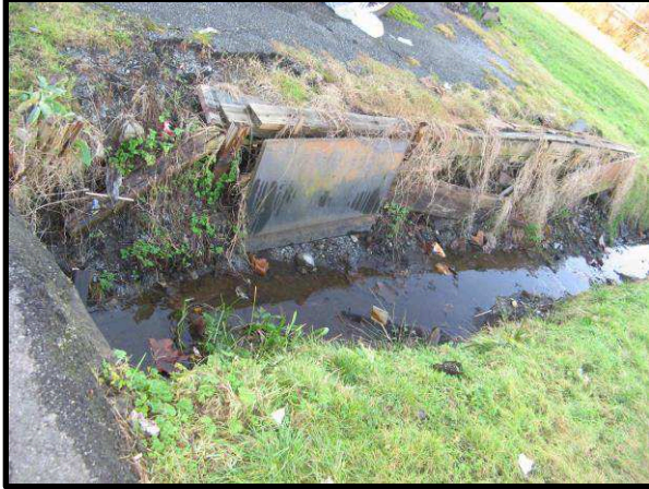
Existing non-standard wroughten wood lining ditch
