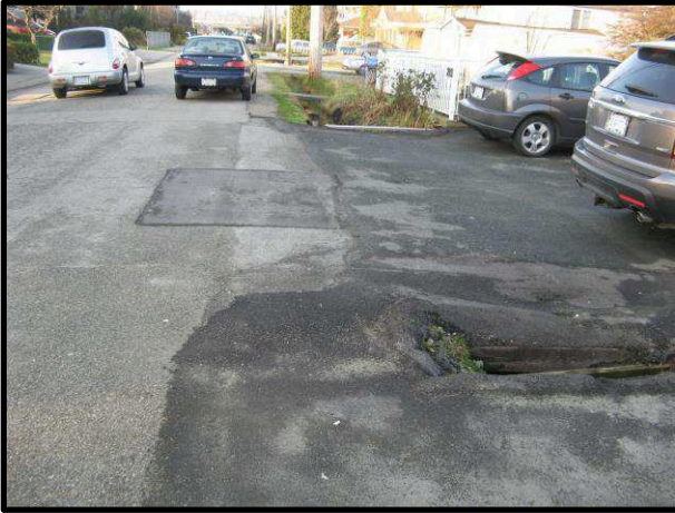
Existing unsafe gap between two driveway culverts
