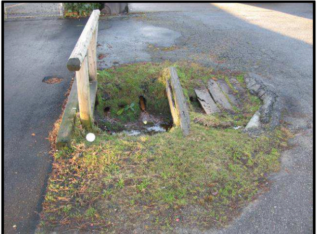
Existing unsightly gap b/n two culverts
