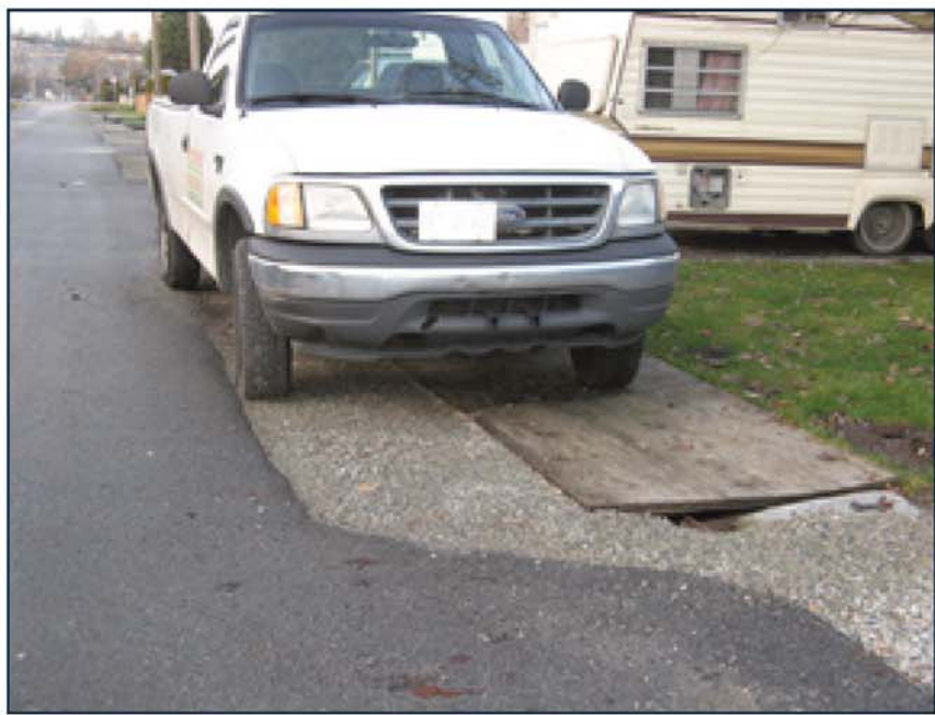
Existing hazardous plywood ditch cover.
