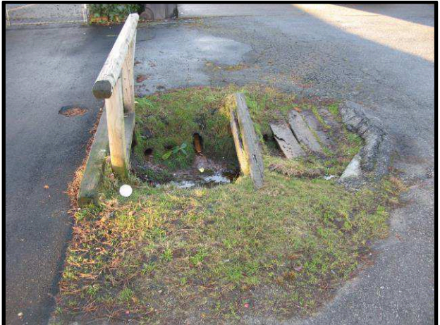
Existing unsightly gap b/n two culverts
