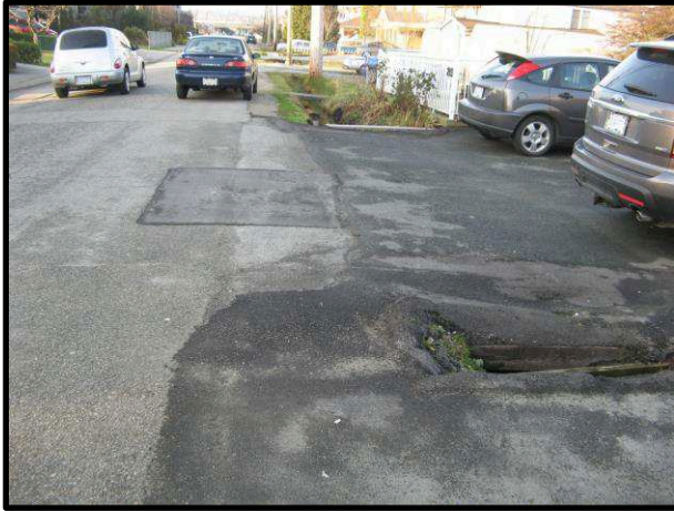
Existing unsafe gap between two driveway culverts
