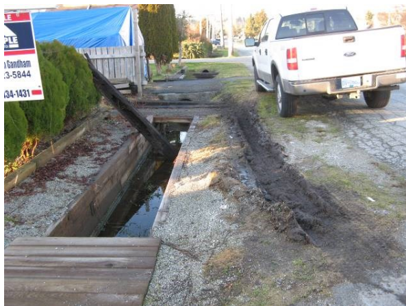
Existing hazardous plywood ditch cover.
