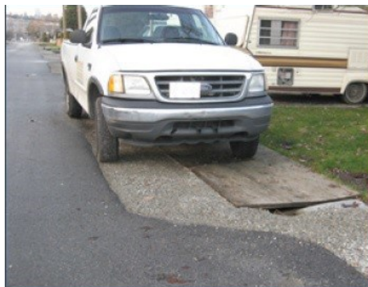
Existing hazardous plywood ditch cover.
