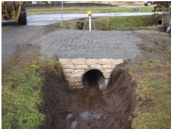
Figure 4 Standard City-installed driveway culvert
