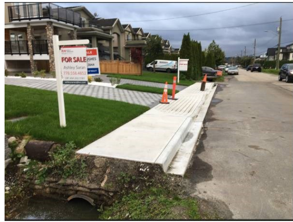
Figure 5 Proper Ditch Enclosure
