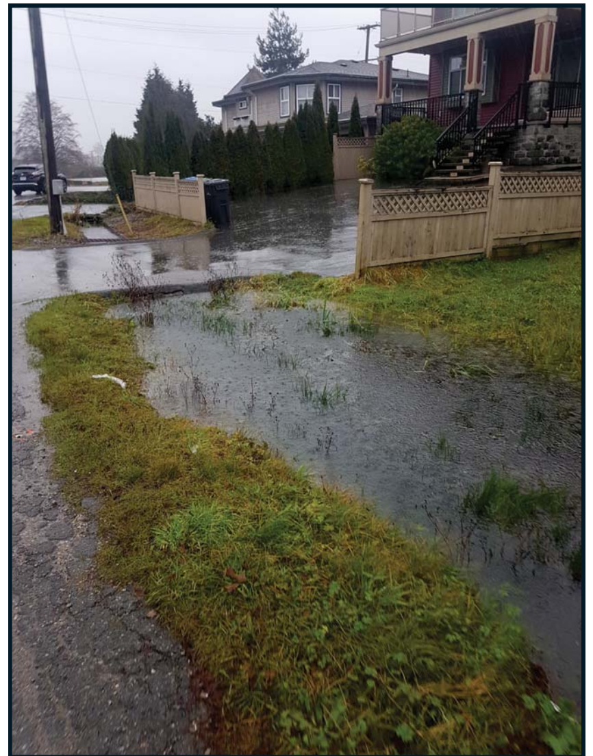
Flooding due to drainage impediments
