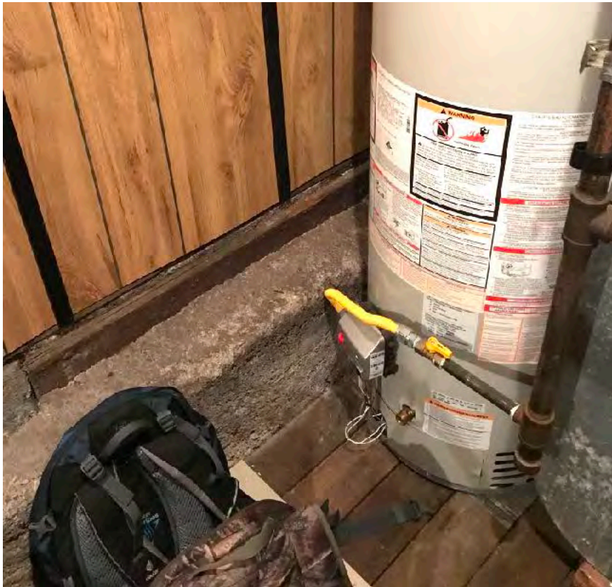
Section of foundation as visible from inside the mechanical room, east side.
