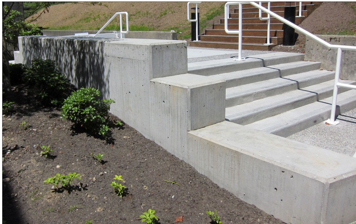
CONCRETE STAIR - SEATWALLS DESCRIPTION: CAST IN PLACE CONCRETE, SANDBLAST FINISH WITH EXPOSED AGGREGATE BAND & HAND RAILS
