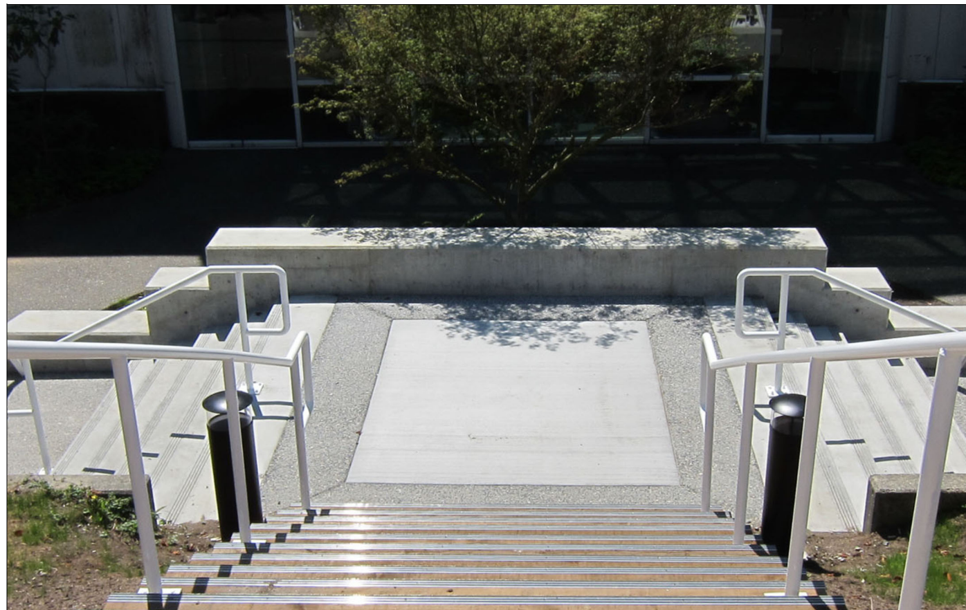
CONCRETE STAIR - LANDING DESCRIPTION: CAST IN PLACE CONCRETE, SANDBLAST FINISH WITH EXPOSED AGGREGATE BAND & HAND RAILS
