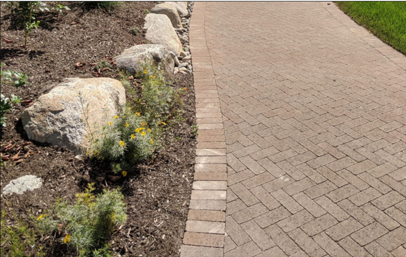
CONCRETE UNIT PAVERS DESCRIPTION: CONCRETE UNIT PAVERS SOLDIER OR HERRINBONE PATTERN
