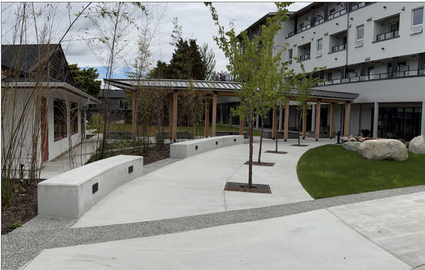
CONCRETE SEATWALL DESCRIPTION: CAST IN PLACE CONCRETE, SANDBLAST FINISH WITH WALL LIGHTING
