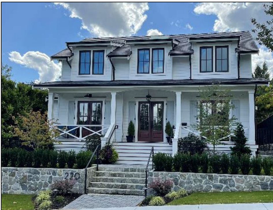
New construction at 220 Second Street
