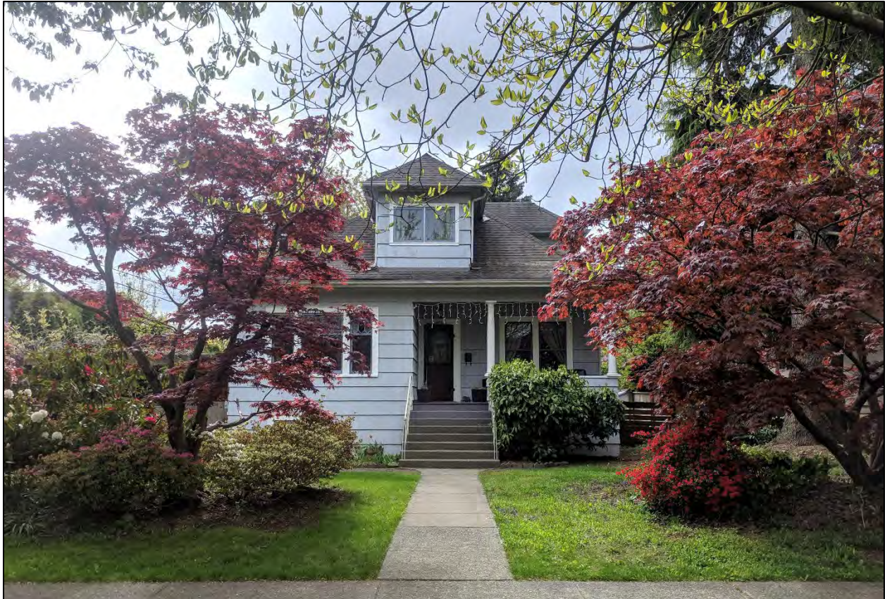
Fig. 1: Calbicks House, 208 Fifth Avenue, New Westminster, BC, 2019. (Source: Cummer)
