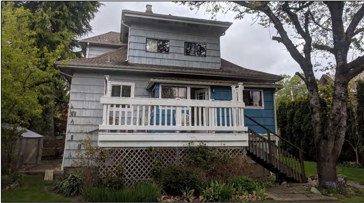
Fig. 10: Back view of Calbicks House at 208 Fifth Avenue, 2019, showing the later addition that will be removed. (Source: Cummer)
