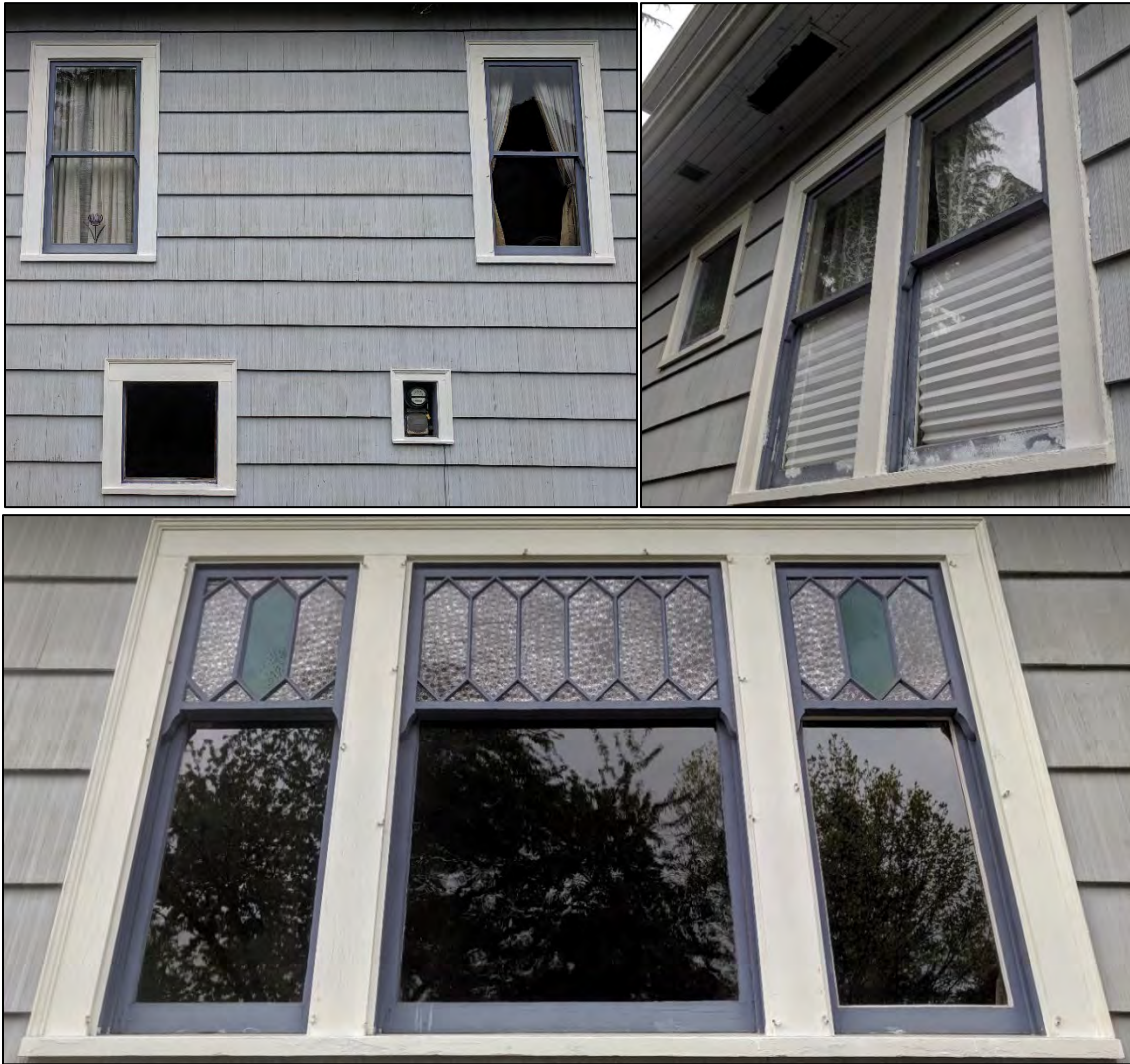
Figs. 22 to 24: Fig. 22 (upper left) shows the eastern side windows of Calbicks House at 208 Fifth Avenue, 2019; Fig. 23 (upper right) shows some of the western side windows; Fig. 24 (bottom) shows the triple window assembly of double-hung horned wood windows with decorative upper sashes at the front of the house. (Source: Cummer)
