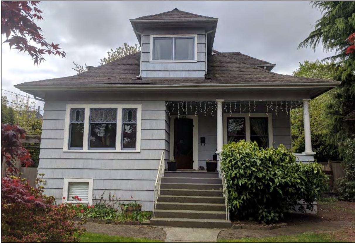
Fig. 8: Front view of Calbicks House at 208 Fifth Avenue, 2019, illustrating the hipped dormer, hipped roof with slight bell-cast flared eaves, the partial-width porch and classical columns, with centred front door. (Source: Cummer)
