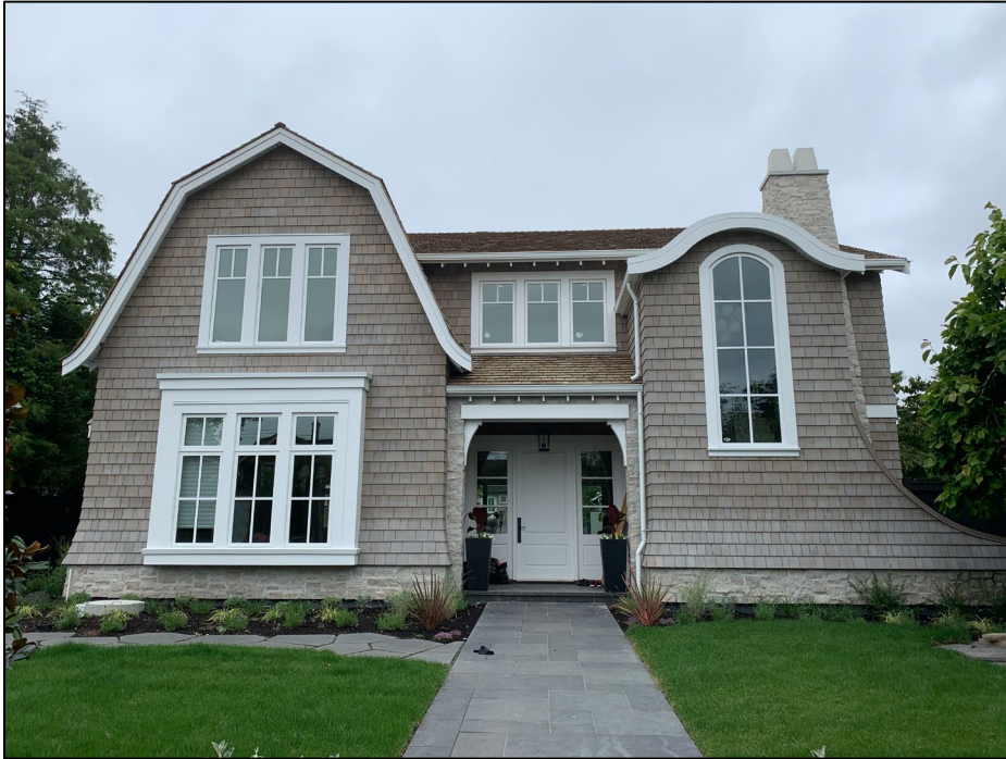
New construction at 217 St. Patrick Street
