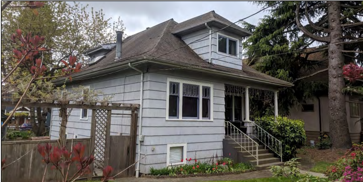
Fig. 9: Partial front and eastern side view of Calbicks House at 208 Fifth Avenue, 2019, highlighting its hipped roof. (Source: Cummer)
