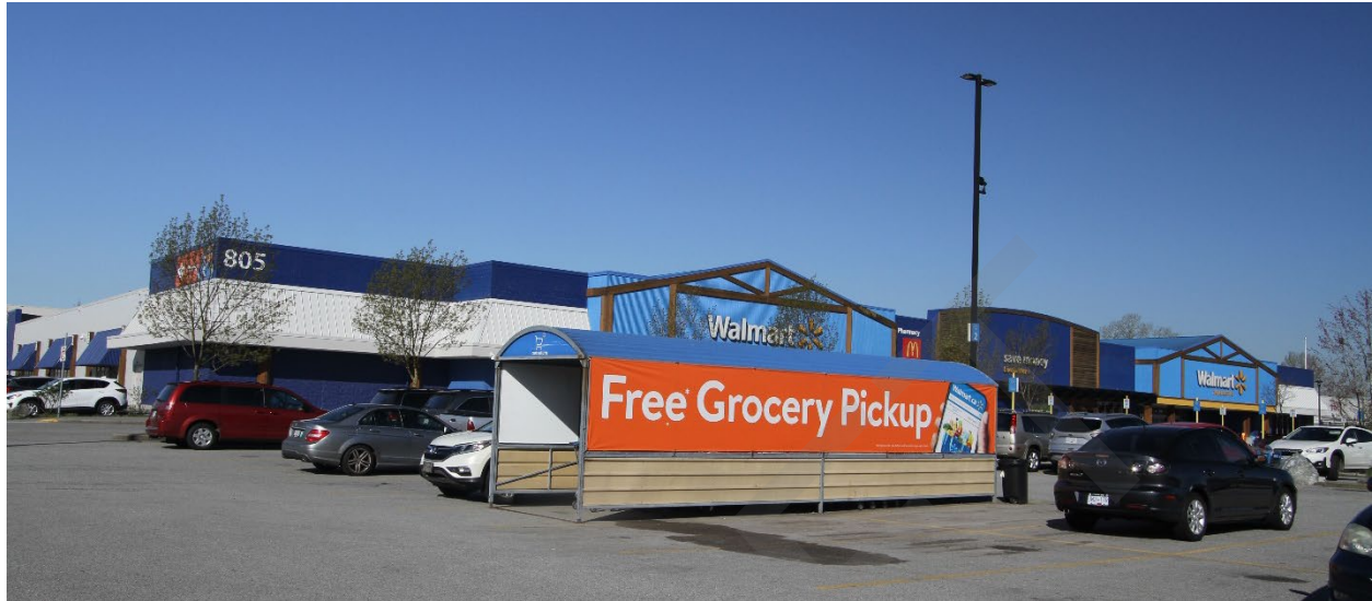
Walmart Supercentre at SmartCentres Queensborough Landing (132,000 sq. ft.)
