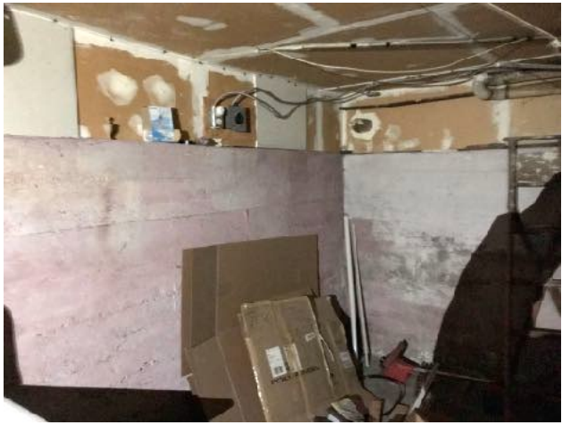
Above: interior (left) and exterior (right) photographs of the board-formed concrete foundation.
