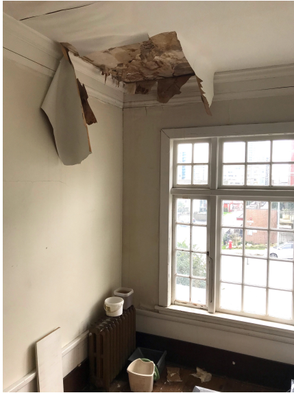
This photo shows water damage in the ceiling in a corner of the main stairway leading to the second floor
