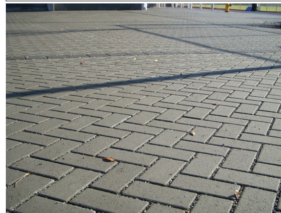
Permeable pavers for driveway
