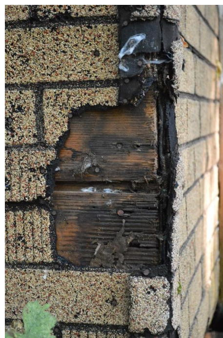
Figure 31: Board underlay beneath insul-brick siding
