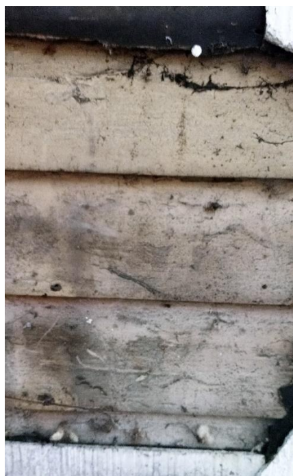
Figure 30: Traces of cove lap siding above the main floor level
