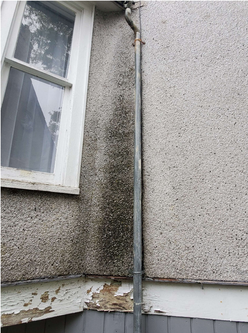
608 long term gutter failure, high chance of structural damage
