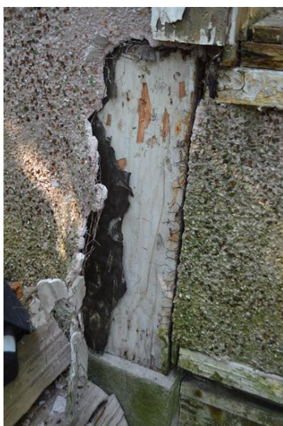
Figure 36: One-inch-thick board underlay beneath bottle dash stucco
