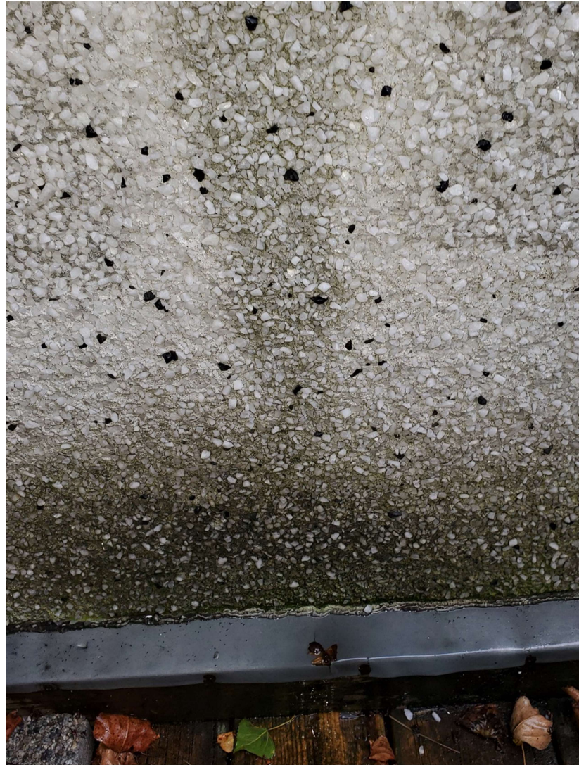
356 long term stucco failure, high chance of structural damage
