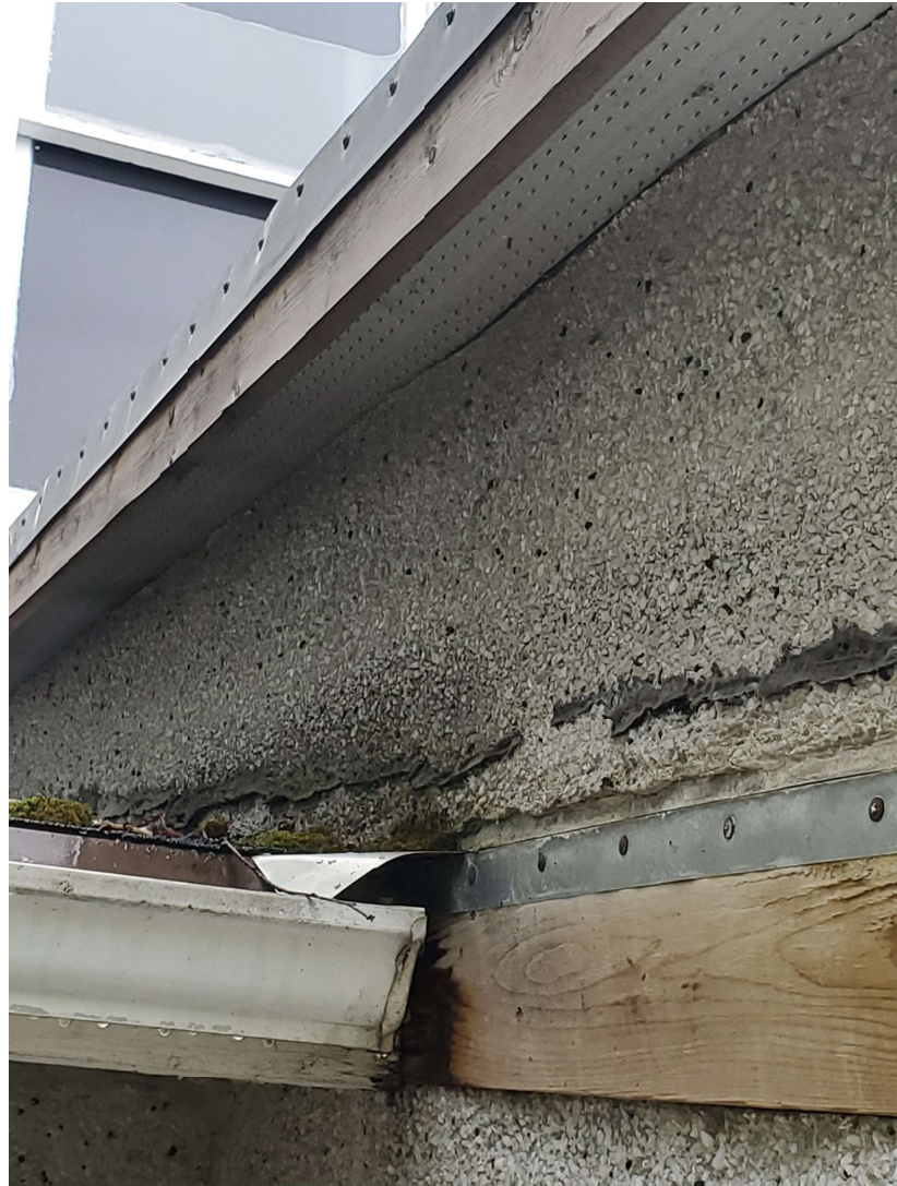
926 poorly maintained roof edges, high chance of internal water damage
