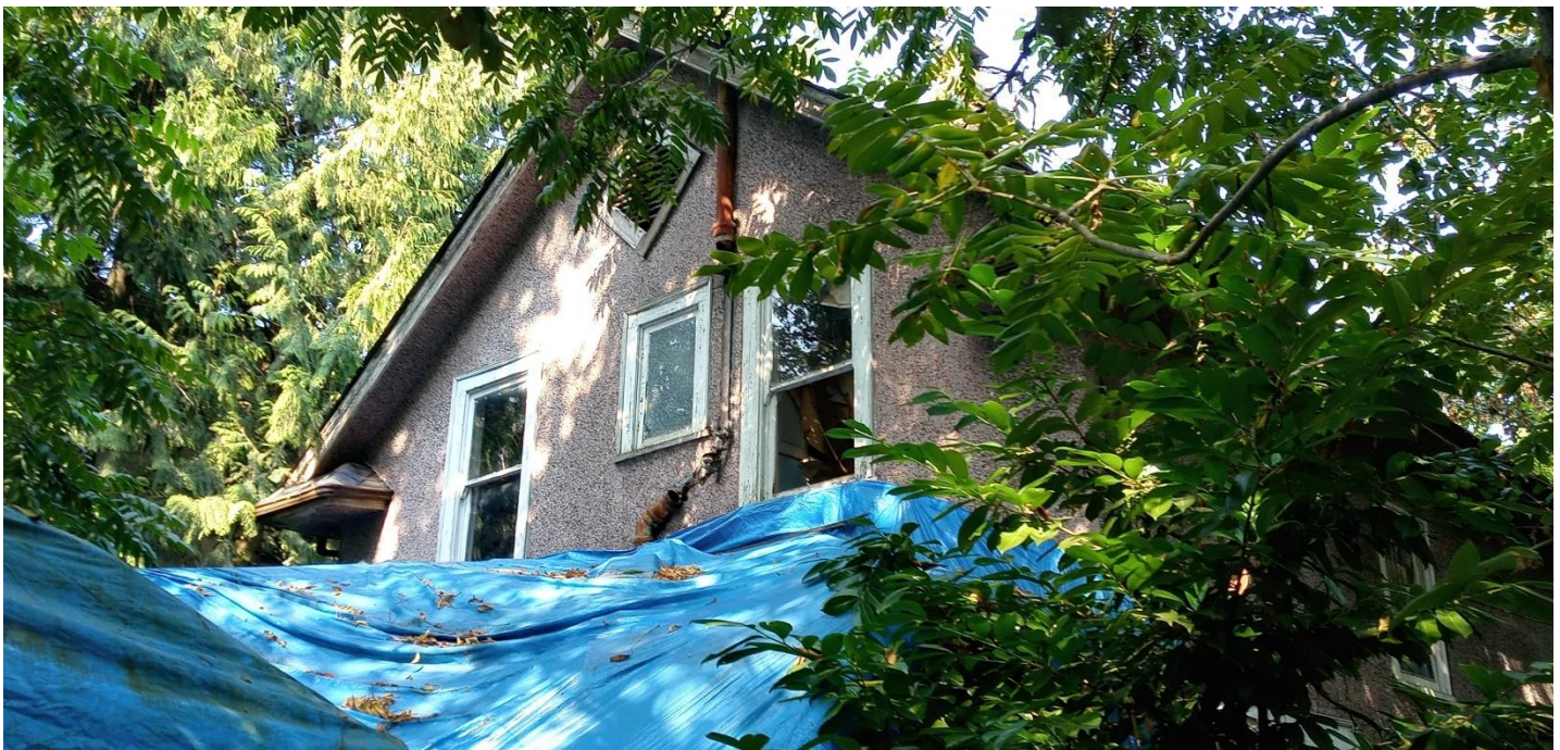
Figure 5: Back elevation with tarp on top of collapsed roof of addition
