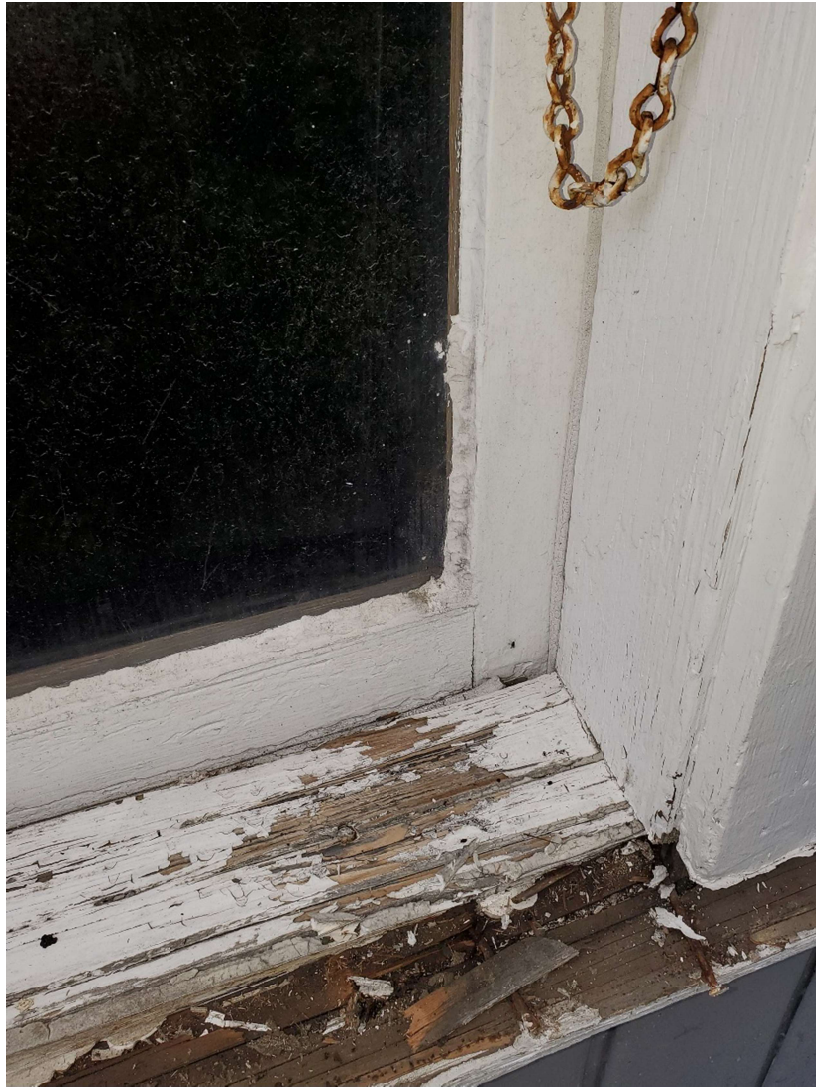
439 most wood windows beyond repair, fully decayed
