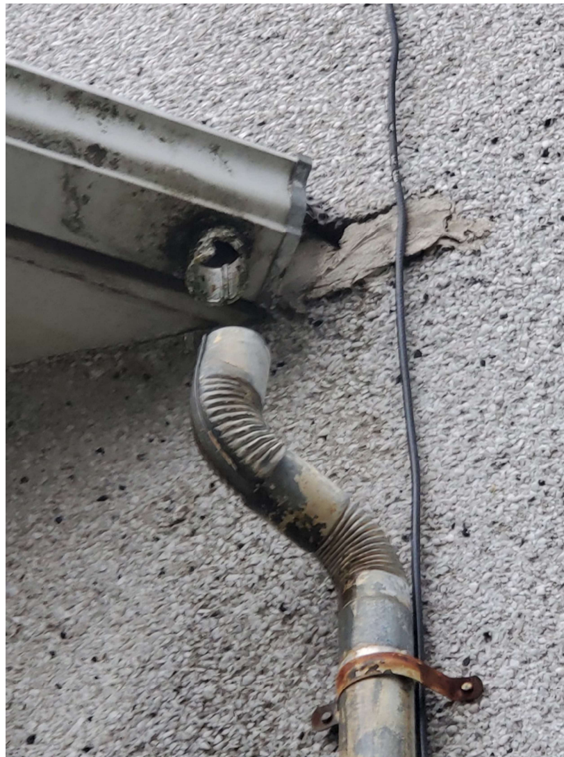
616 Long term gutter and stucco failure, high chance of internal rot and mold
