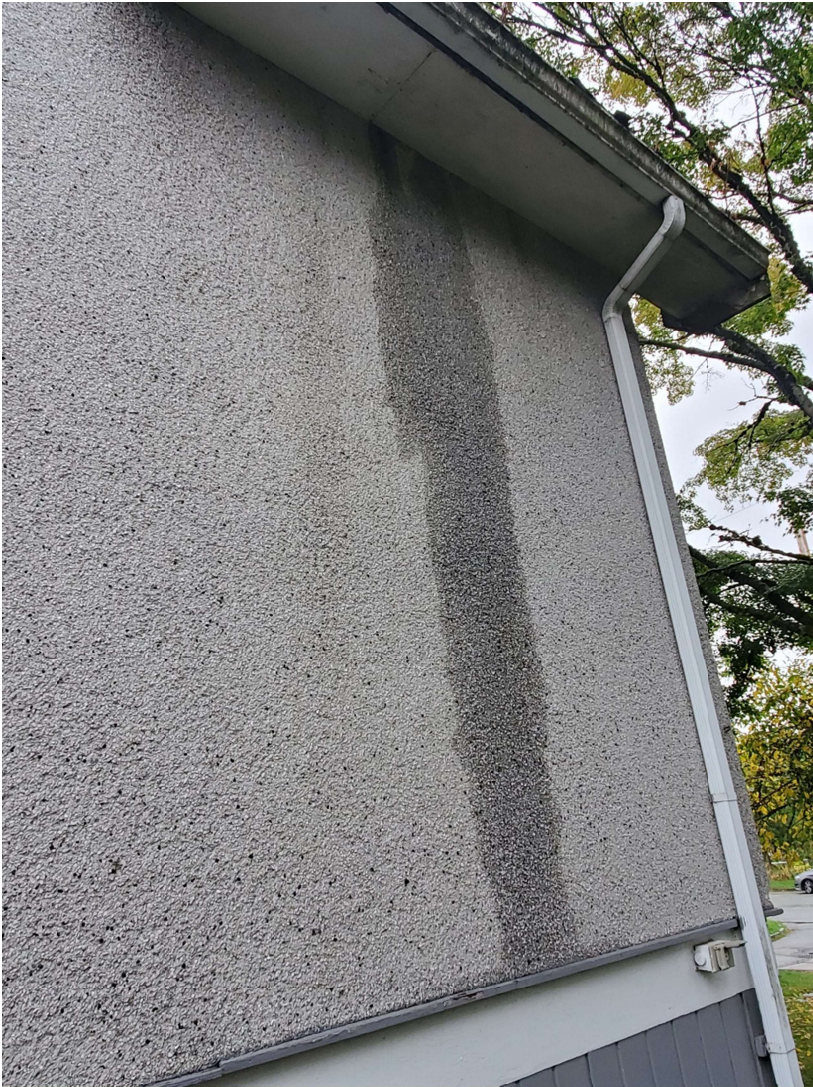
621 roof failure, high chance of structural damage
