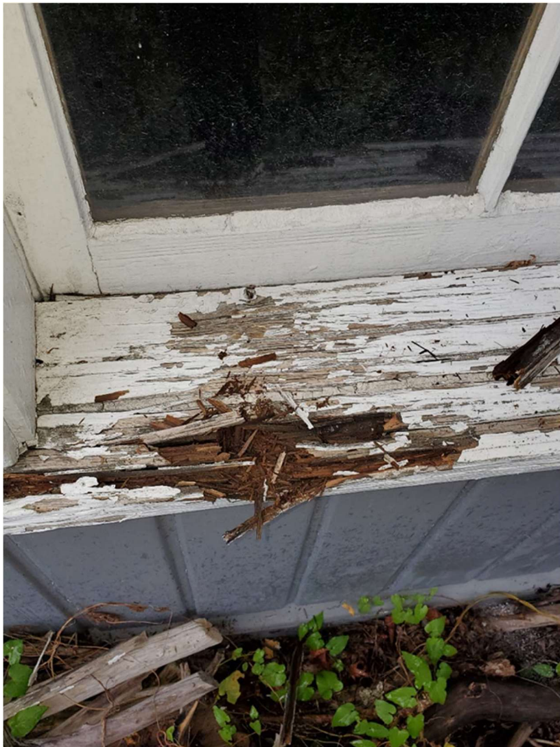
416 most wood windows beyond repair, fully decayed
