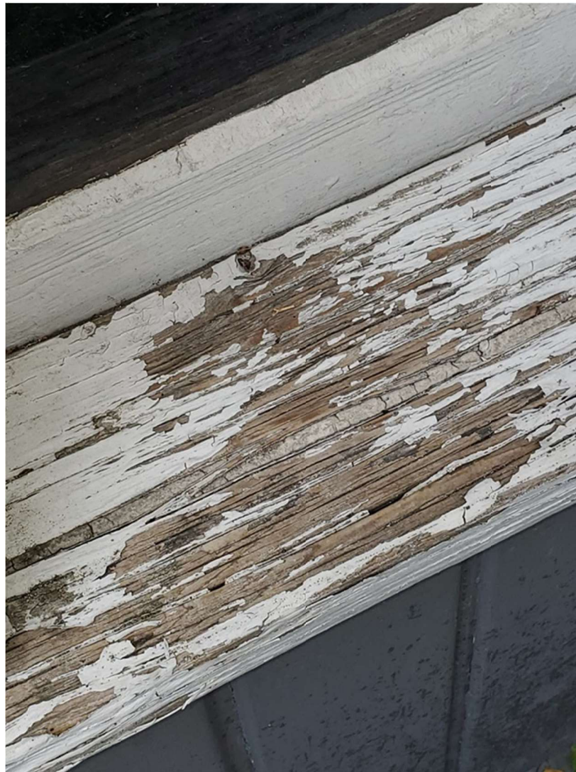
503 most wood windows beyond repair, fully decayed
